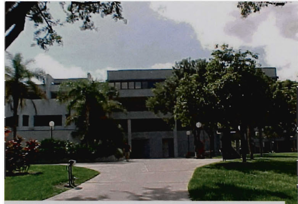
Fig.B.16- View of Deuxieme Maison (DM) from central campus courtyard
