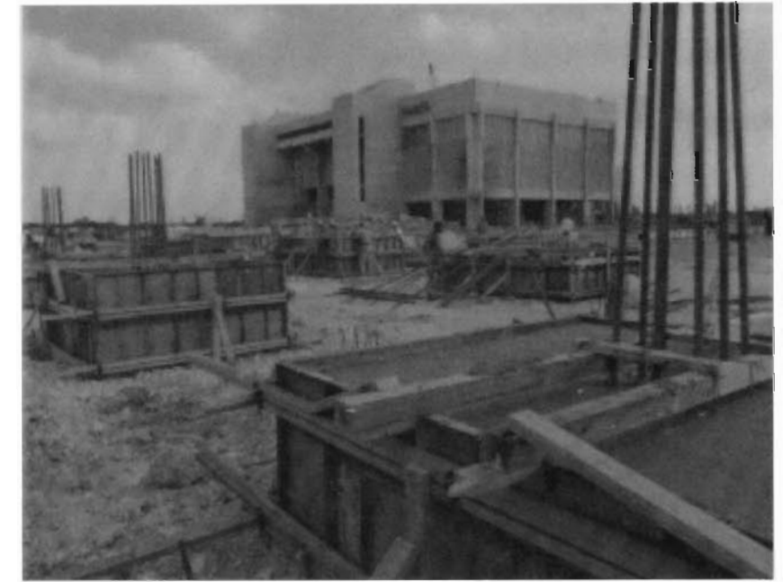
Fig.B.13- Deuxieme Maison (DM) building, overlooking construction site in 1973.
