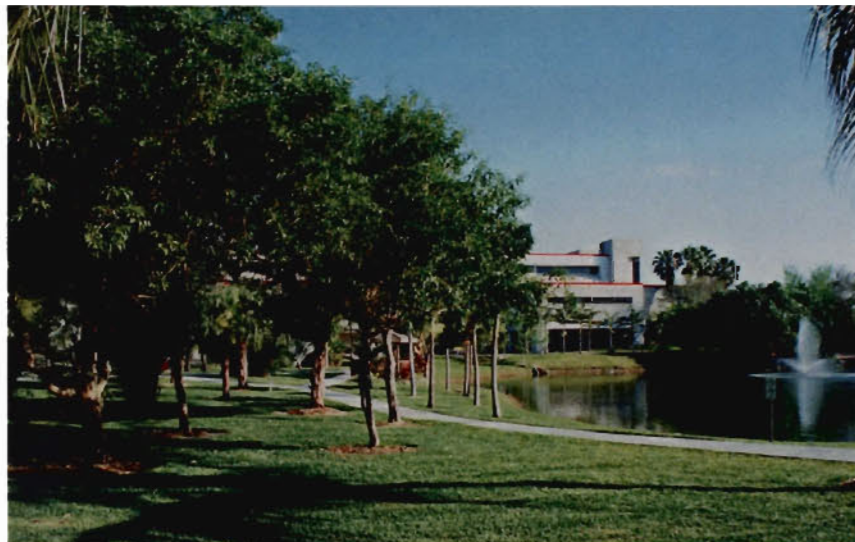
Fig.B.26- Facing north toward ECS building. Building built in 1989
