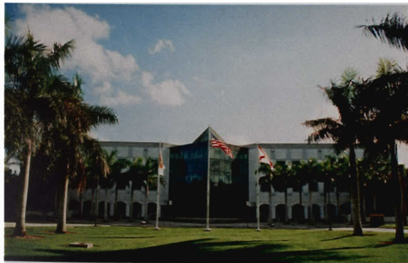
Fig.C.15- view of Business Building (BA) facing the mall
