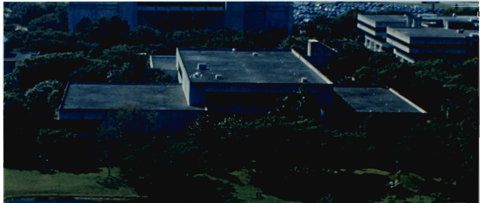
Fig.B.14- Aerial view of the old library building built in 1975 (c. 1988).
