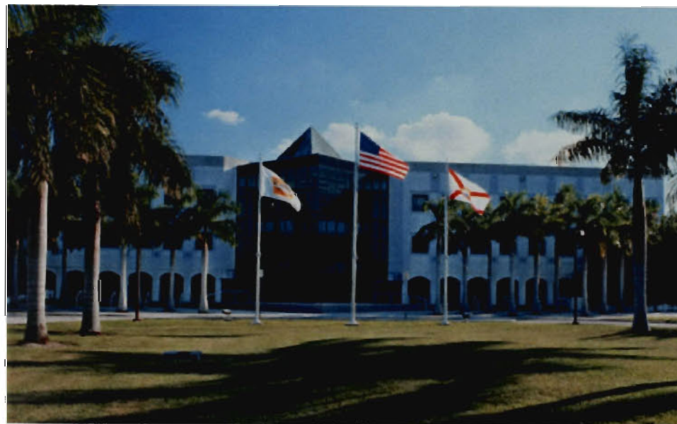
Fig.B.29- View of Business Building, built in 1992.
