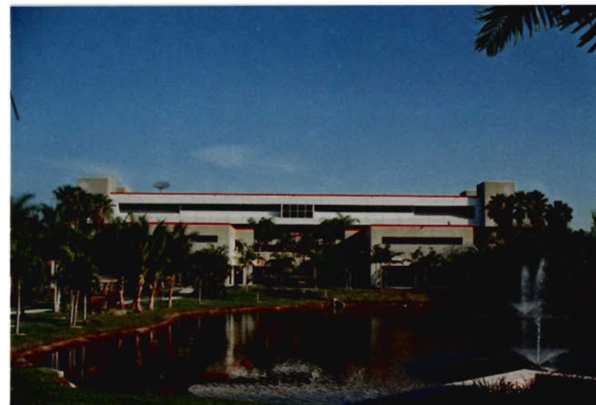
Fig.C.13- View of south elevation of ECS building facing lake area
