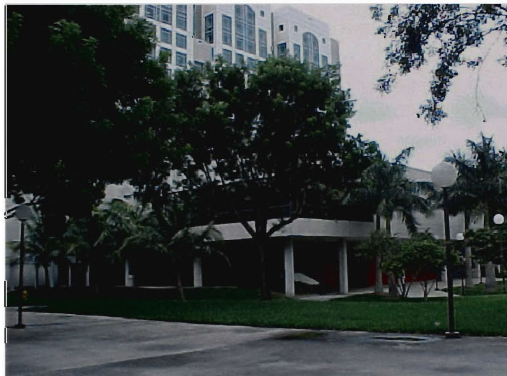
Fig.B.17- View of the original library from central core (tower behind)
