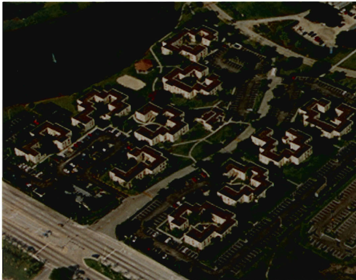
Fig.B.21- Aerial view of dorms along S.W. 107 th Street. Dormitories built in 1985 (c.1994).
