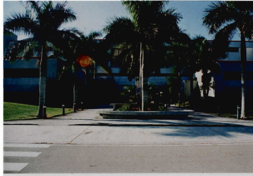
Fig.C.11- View of formal Entrance to the Engineering & Computer Science Building (ECS)
