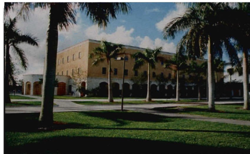
Fig.C.17- View of east elevation of the Education Building (COE) facing mall
