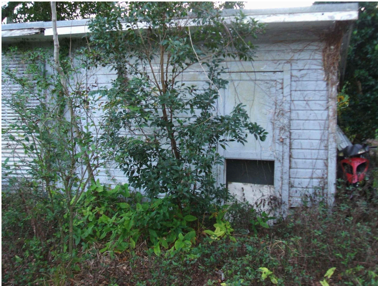
Pump house and storage
