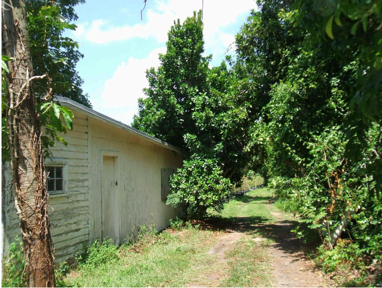
Pump house and storage
