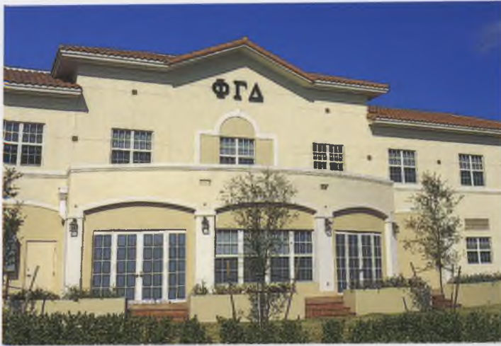
The completion of the Phi Gamma Delta House, FIU's first fraternity house, marked the start of what eventually will become "Fraternity Row."
