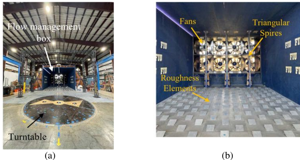
Figure 3.1. (a) Inside the FIU Wall of Wind (WOW) Experimental Facility (EF), (b) The flow management box with roughness elements and spires for generating the desired ABL
