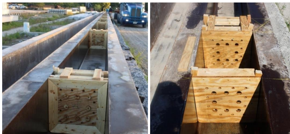
Figure 46: Wooden headers arrangement in casting bed
