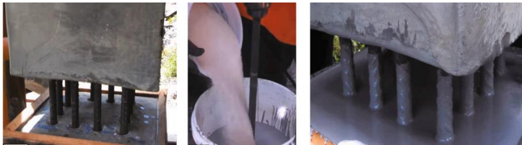
Figure 15: An example of dowel-type splice for PPCPs [40]
