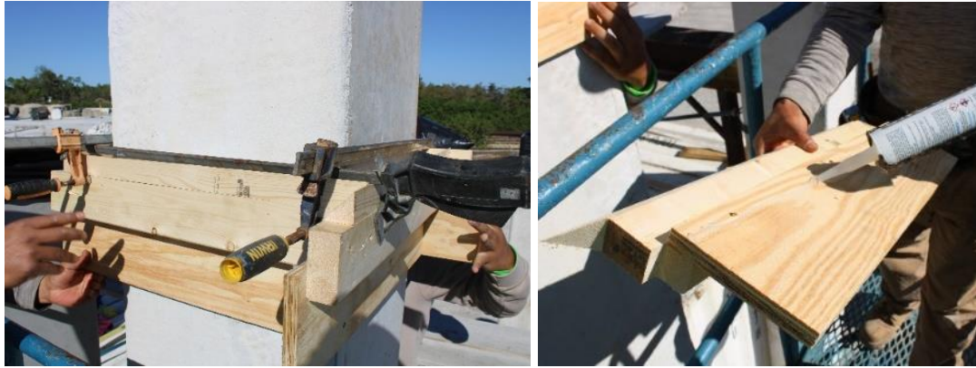
Figure 60: Wooden framework used for splicing the pile specimens
