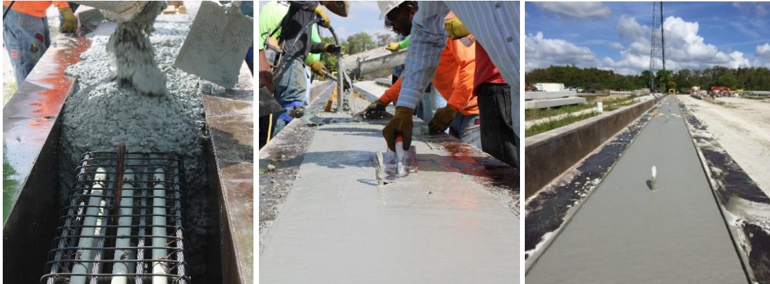
Figure 55: Casting concrete
