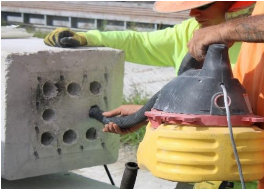
Figure 58: Drilling (top) and cleaning (bottom) the holes for Unforseen Splice specimens
