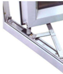
Figure 2.2: Extender type hinge
