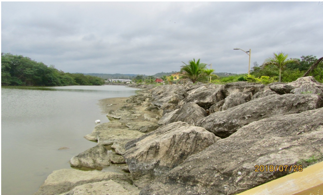
Figure 11. Manglaralto river wall. Source: The author (2018)
