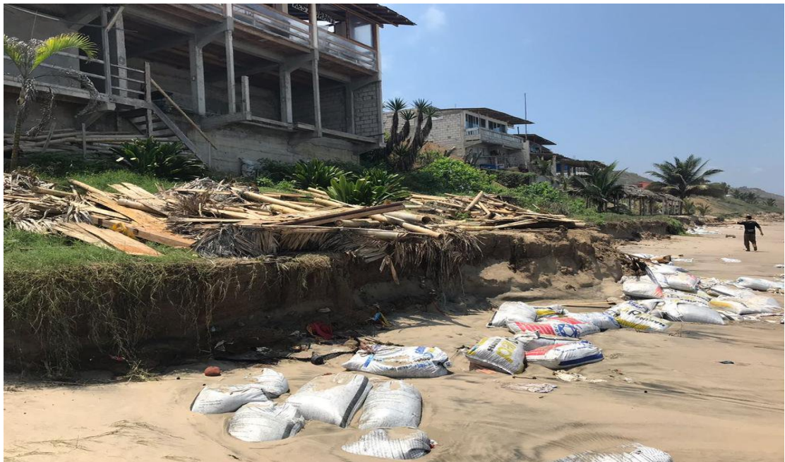
Figure 14. Damages at Libertador Bolívar south beach during September 2018. Source: El Universo (2018)
