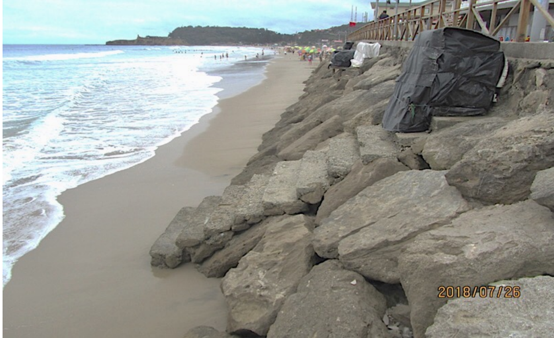
Figure 8. Seawall at Comuna Montañita. Source: Author (2018)
