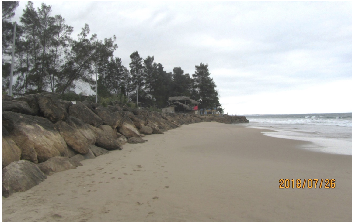
Figure 9. Seawall at Comuna Manglaralto. Source: author (2018)
