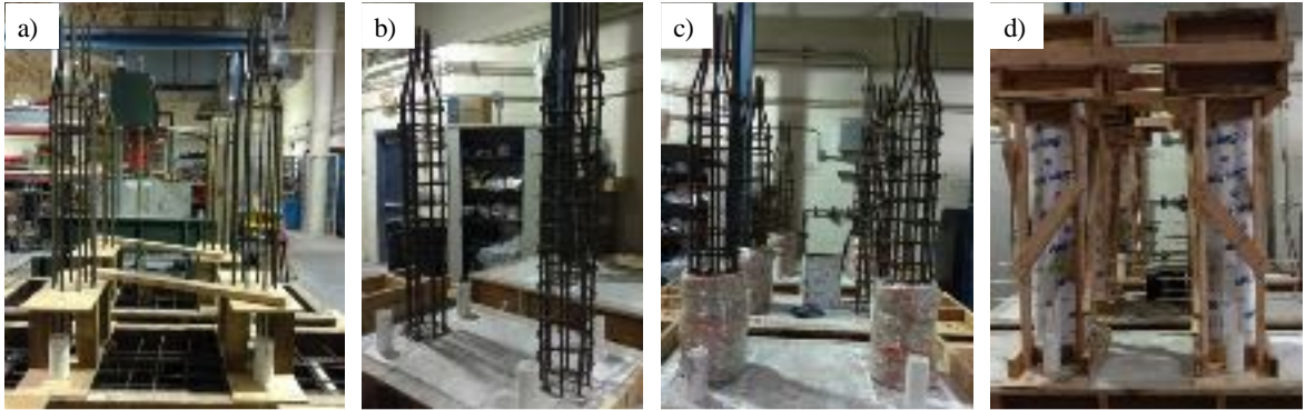
Figure 4- 2 The construction process of a typical specimen: a) formwork and caging, b) casting the footing, c) simulating the damage, and d) erecting the columns, and casting the concrete substrate.
