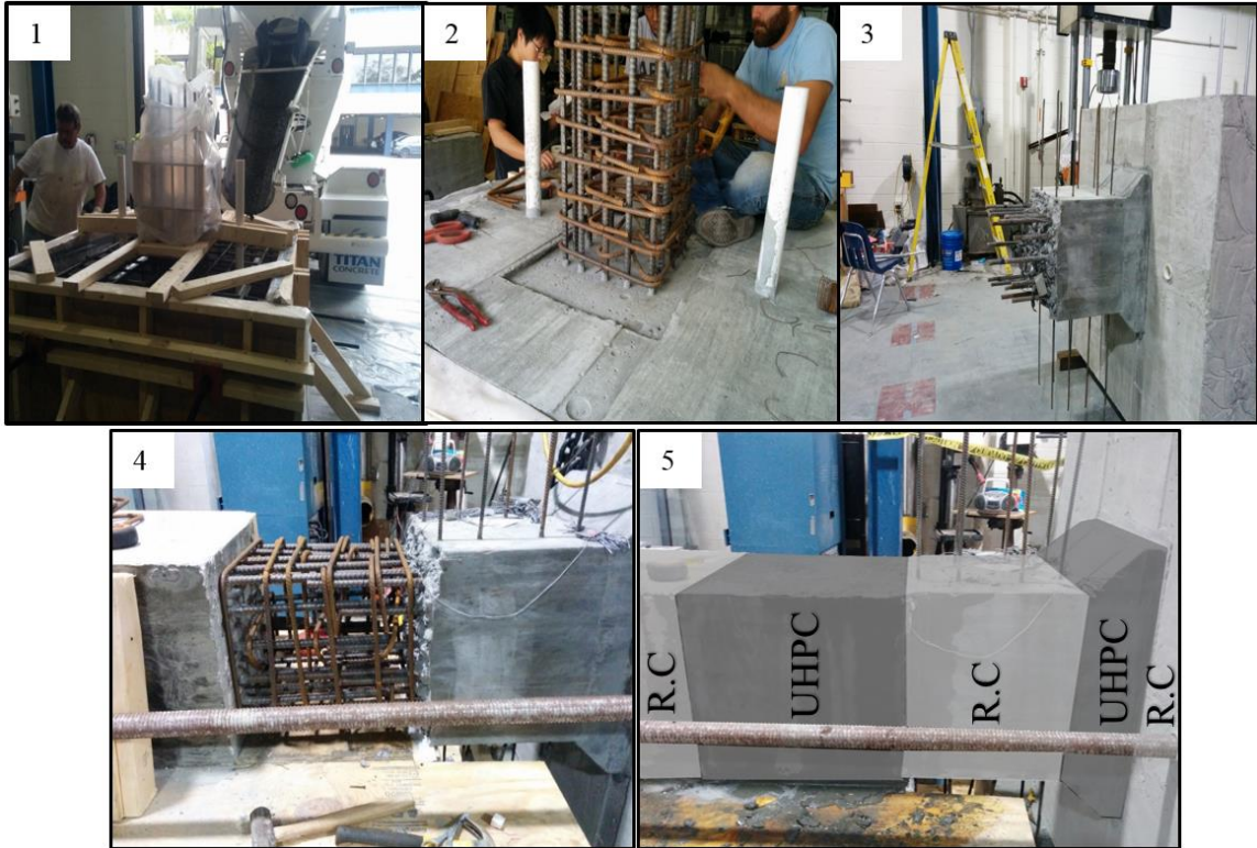
Figure 4-4 Specimen construction procedures.
