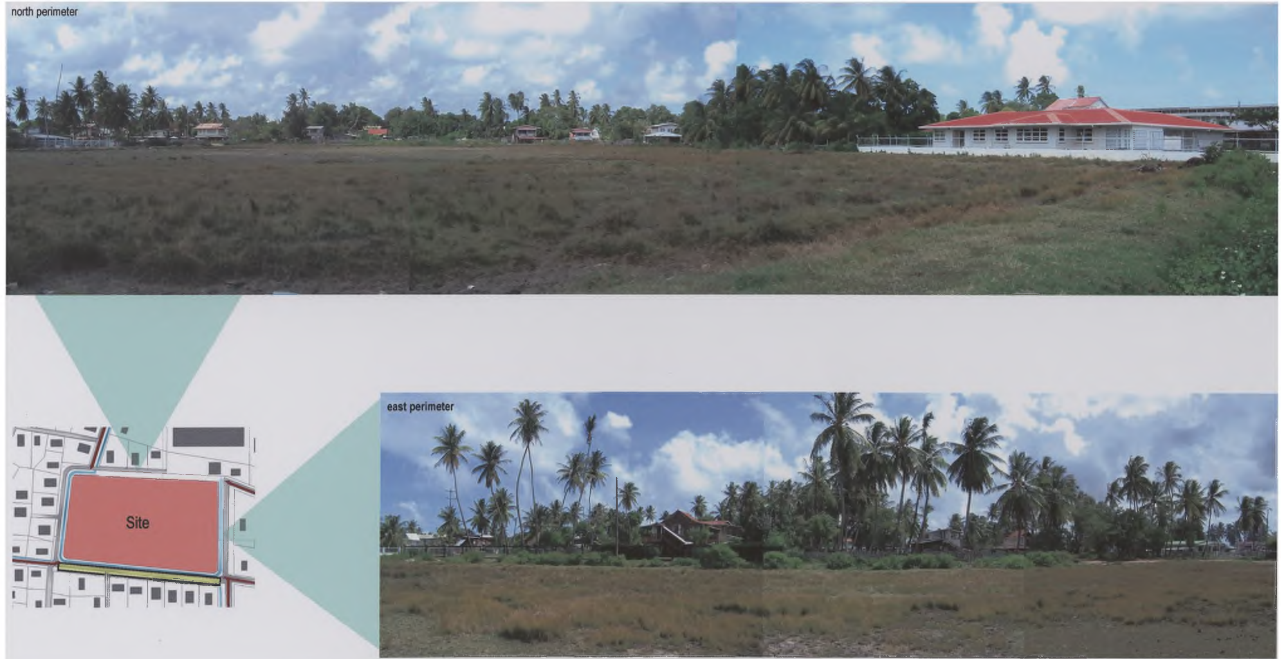
Figure 32: North Perimeter (above), East Perimeter (right)
