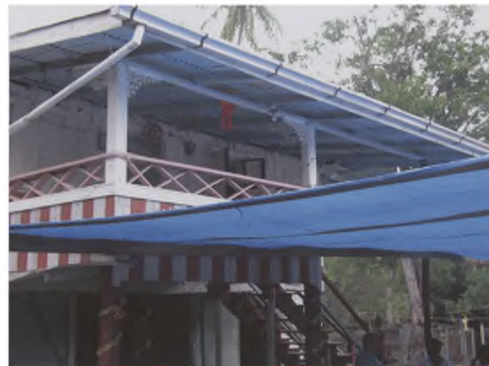
Figure 15a: Jagan House: Large Social Gathering. A temporary structure of wood and canvas extends the bottom-house space.
