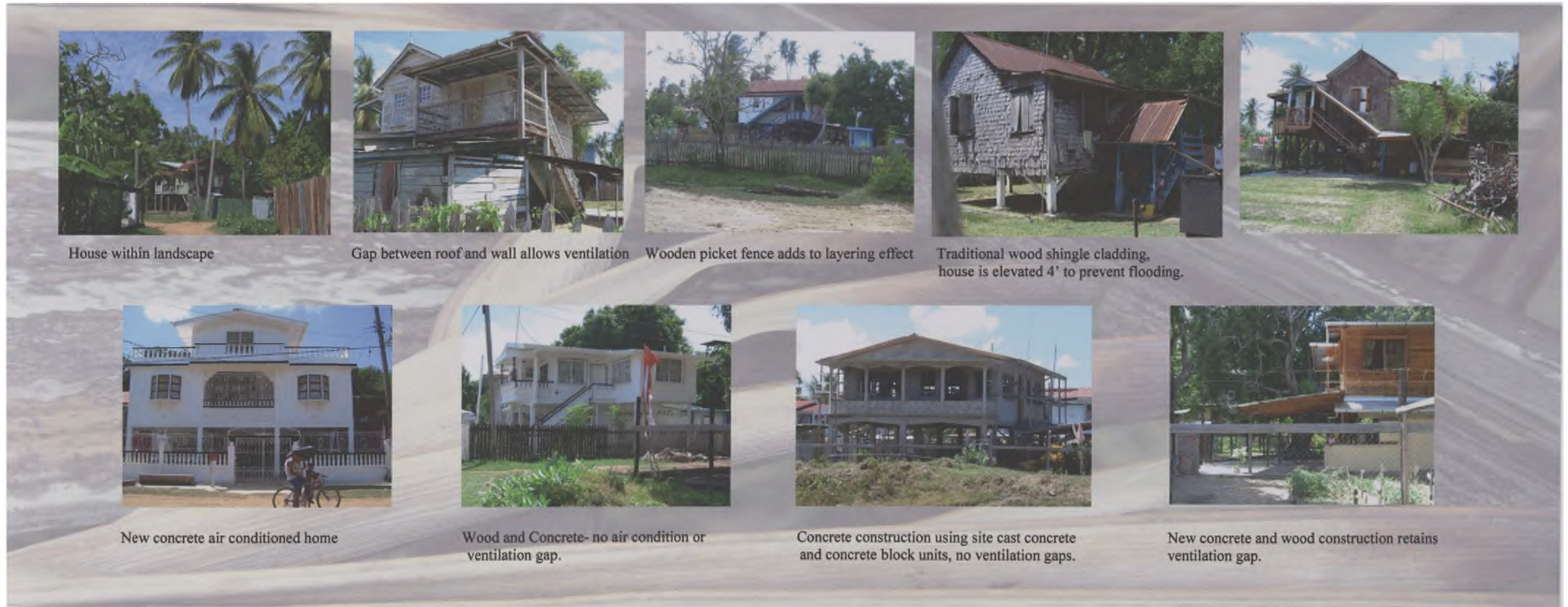
Figure 23: Ankerville, Port Maurant—Traditional Housing (above) Figure 24: Ankerville, Port Maurant—New Housing (below)
