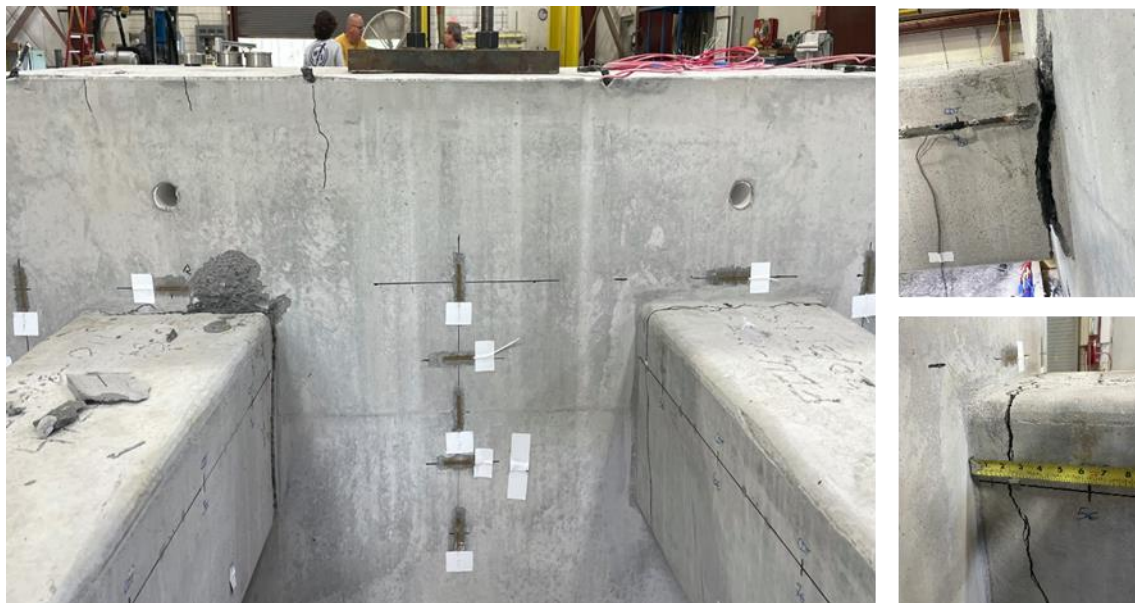
Figure D.54: SP-04 failure mechanism
