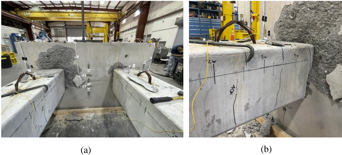
Figure D.130 : SP-08 failure mechanism (a) pile crushing (b) cracks in pile
