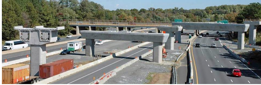
Figure 3.44: Straddle bent (courtesy of Corven Engineering)
