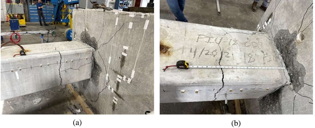
Figure 5.89: Photographs of the failure of SP-03
