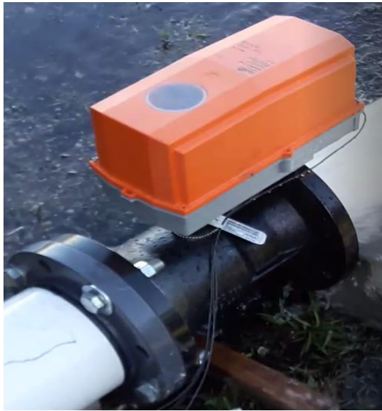
Figure A-1: Actuated Ball Valve
