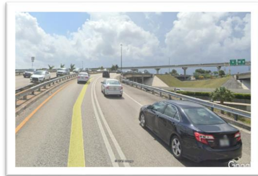
Paved with Guardrail
