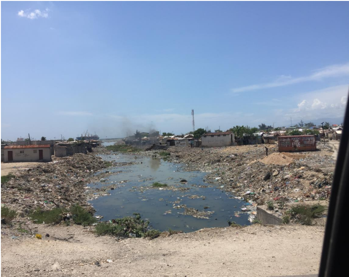
Figure 7.1: Drainage filled with debris and trash near Cité Soleil 32 .
