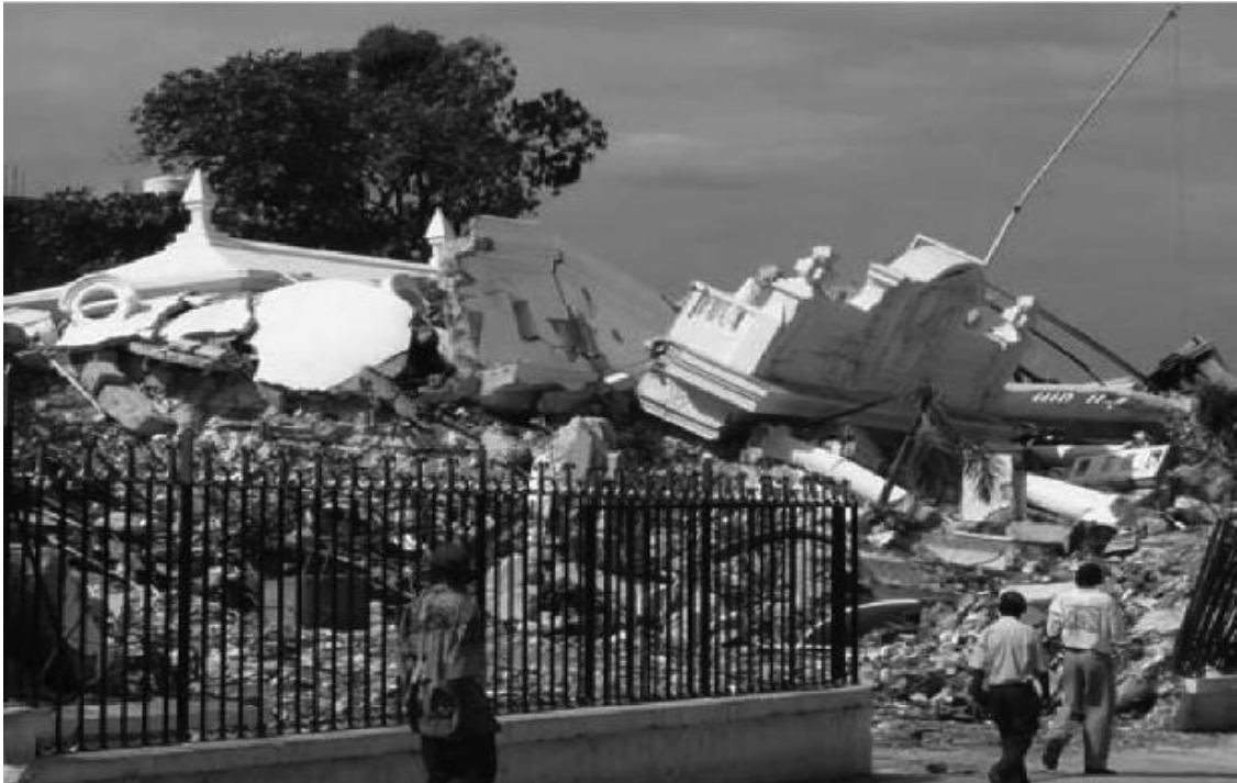
Figure 6.2: Palais de Justice (Justice Palace) in Haiti after the earthquake
