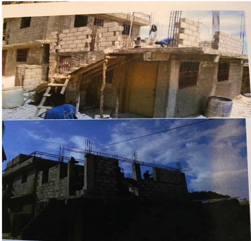
Figure 7.2: Homes built by GOAL in Turgeau, Port-au-Prince
