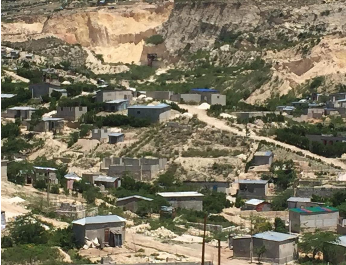
Figure 6.7: Photo exposing the risk of a landslide in Canaan 20 .
