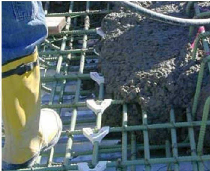
Figure 2-35: Bridge installation of smart aggregate in holders [35]
