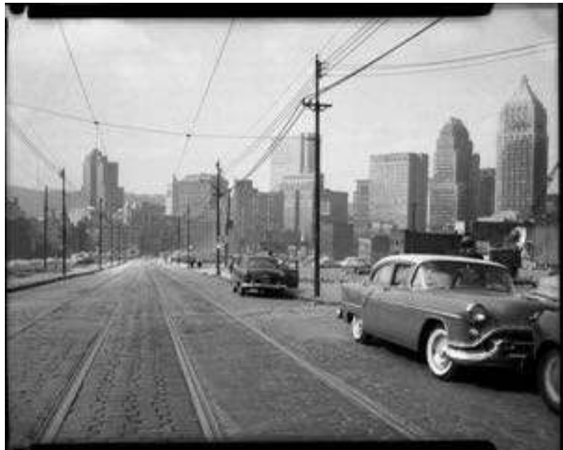
Figure 5.23: Hill District looking toward downtown after demolition. Demolition area from Wylie Avenue near Townsend Street, toward Downtown, Hill District, c. 1955-1957. Courtesy of Carnegie Museum of Art, Charles “Teenie” Harris Archive. Accession number: 2001.35.3439.
