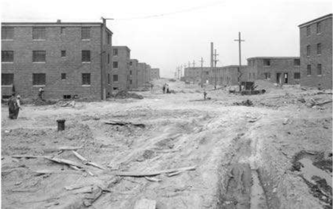
Figure 5.2: Construction of the Bedford Dwellings, May 23, 1940. Pittsburgh City Photographer Collection. 715.4055959.CP.
