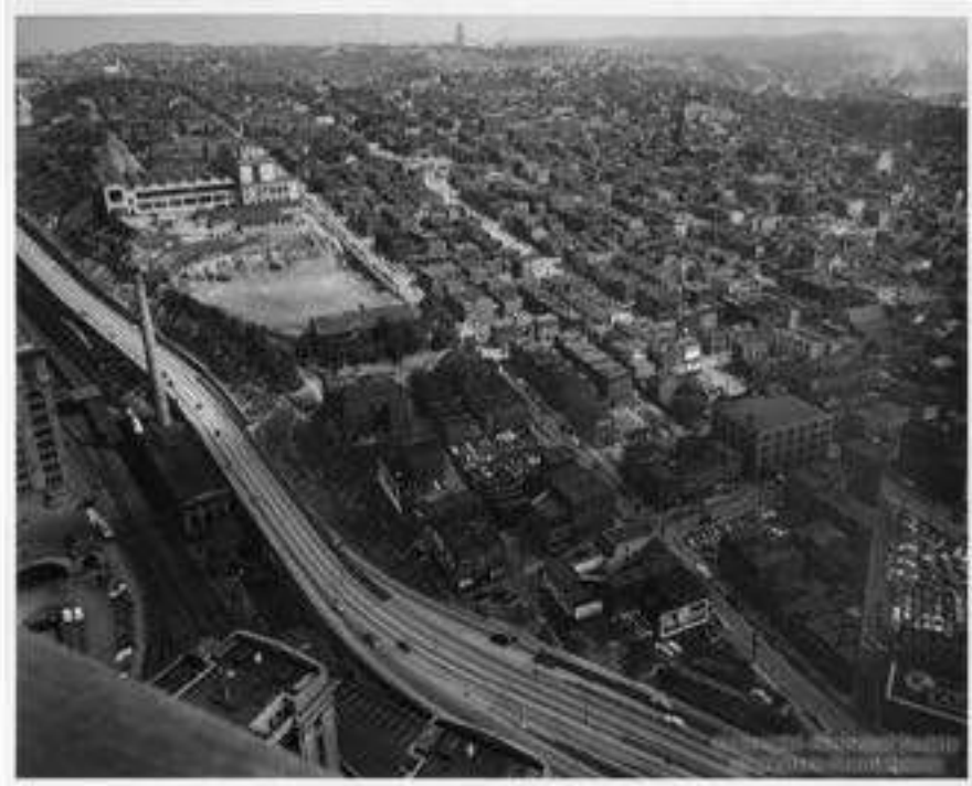
Figure 5.24: Lower Hill District before demolition. Allegheny Conference on Community Development Photographs, MSP285.B033.F04.I02.
