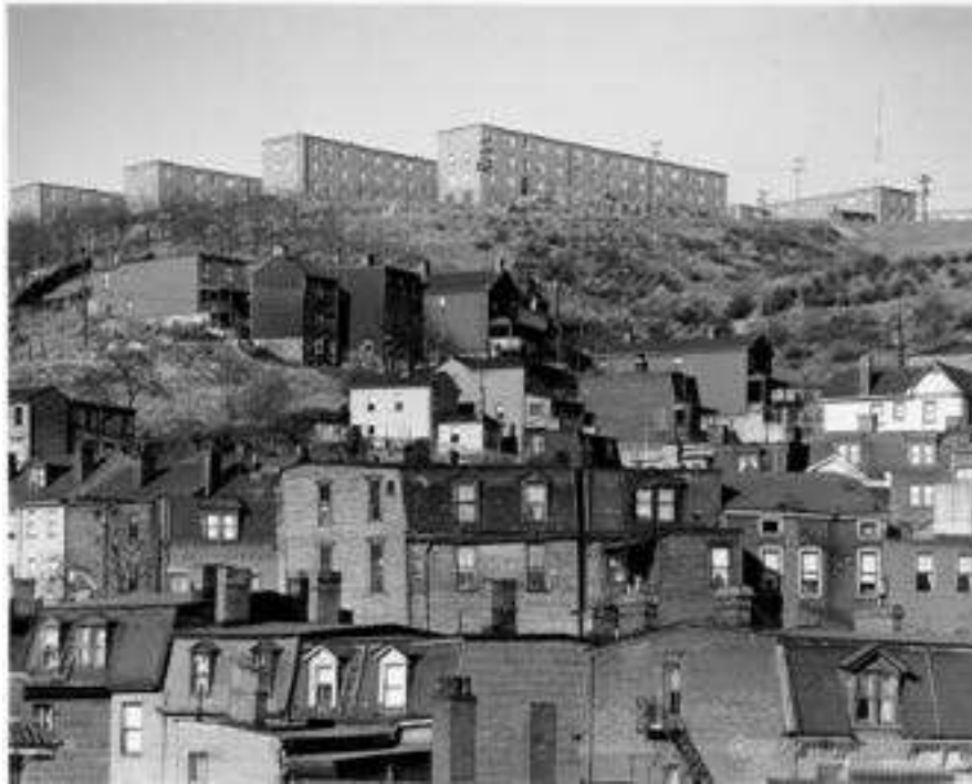
Figure 5.3: Terrace Village public housing complex sitting atop a hill. Allegheny Conference on Community Development Photographs. MSP285.B012.F15.I14.
