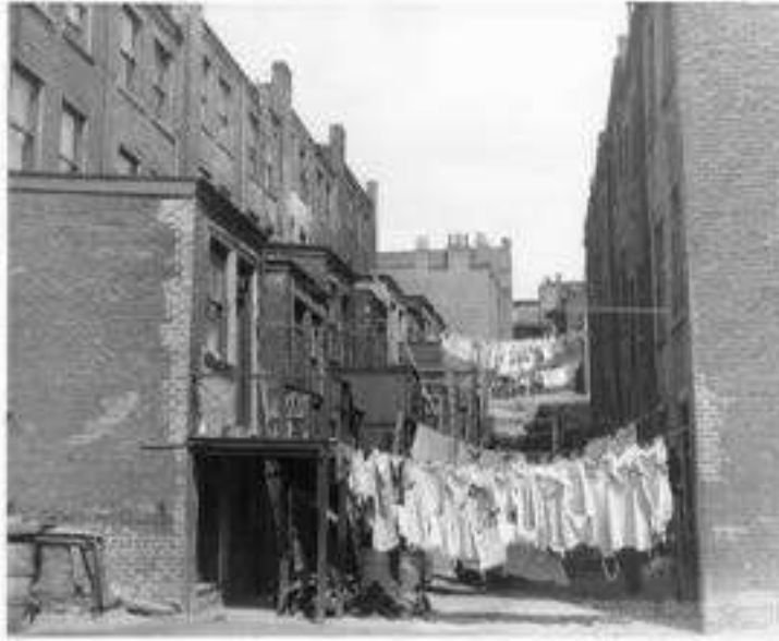
Figure 5.14: Scenes of the Lower Hill before demolition taken by photographer for Allegheny Conference on Community Development, circa 1954. Allegheny Conference on Community Development Photographs, MSP285.B033.F06.I01.
