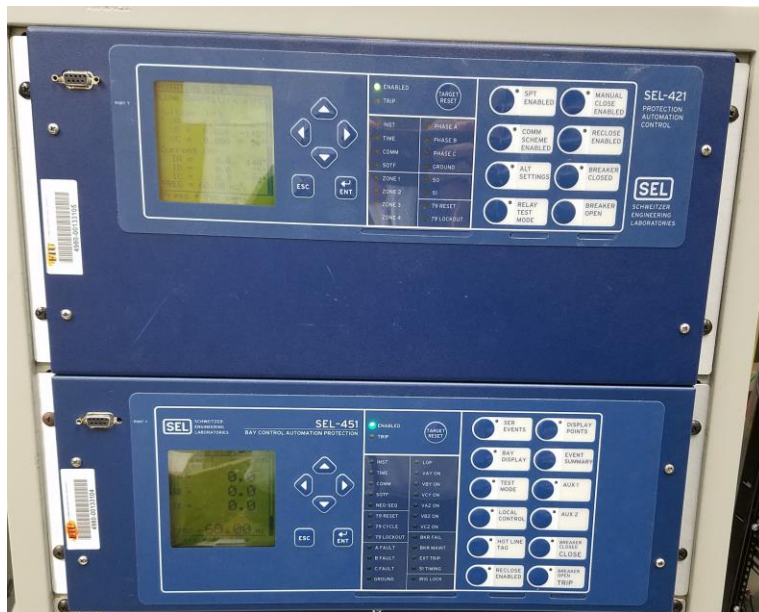
Figure 2.8 SEL Phasor Measurement Units.
