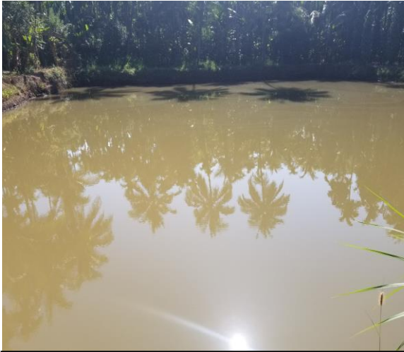
(c) Keresara tank exhibits levels of high siltation and debris buildup, decreasing its potential for water storage
