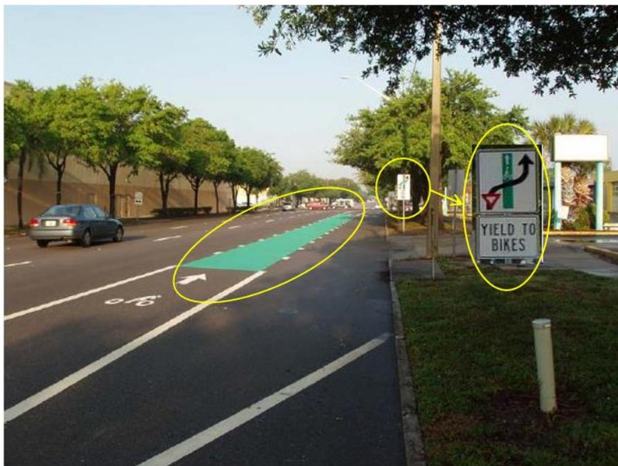
**Figure 2-3: Green-colored Pavement and Accompanying Signing in a Bicycle Lane Weaving Area in St. Petersburg, FL (Source: Hunter et al., 2008)**
