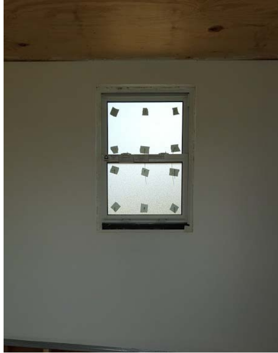
Figure 47. Interior of the building model
