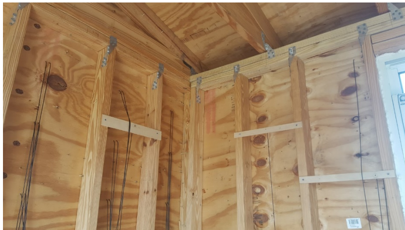
Figure 46. Wall with wood studs
