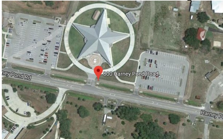
Figure 7.9 Aerial View of Seminole Veterans Building
