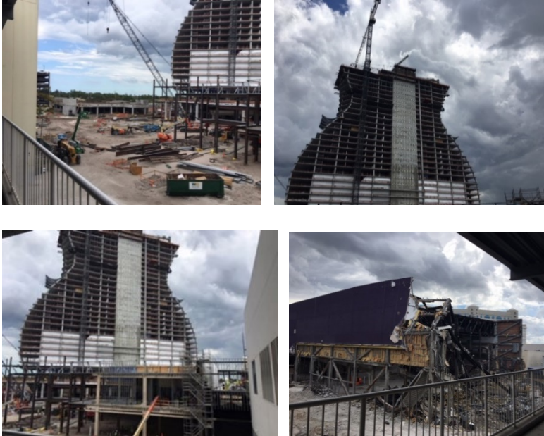
Figures 5.17–5.20 Construction of Hard Rock Hollywood
