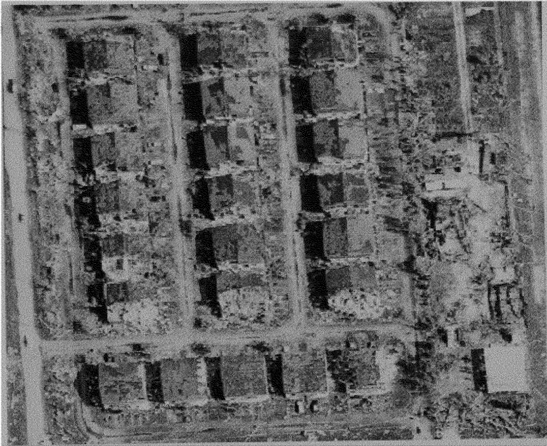
Figure 1.3. Progressive roof cover damage.
