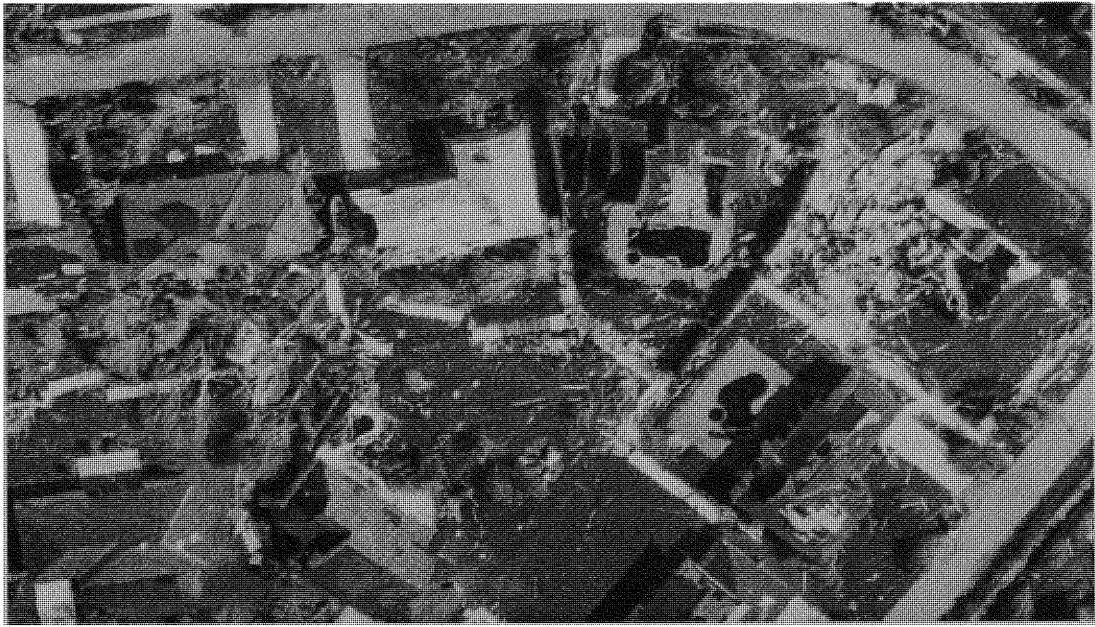
Figure 1.20. Failure occurred due to development of suction force.
