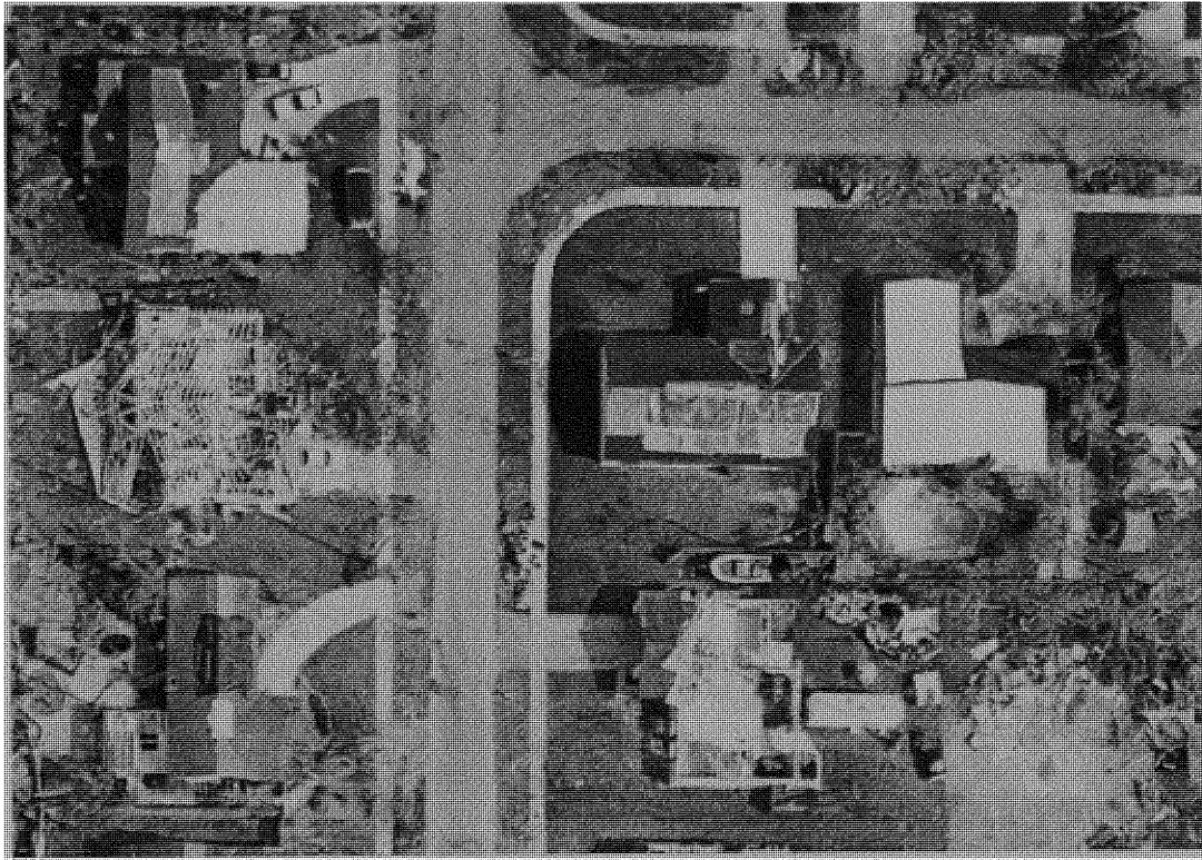
Figure 1.6. Variable roof system damage.
