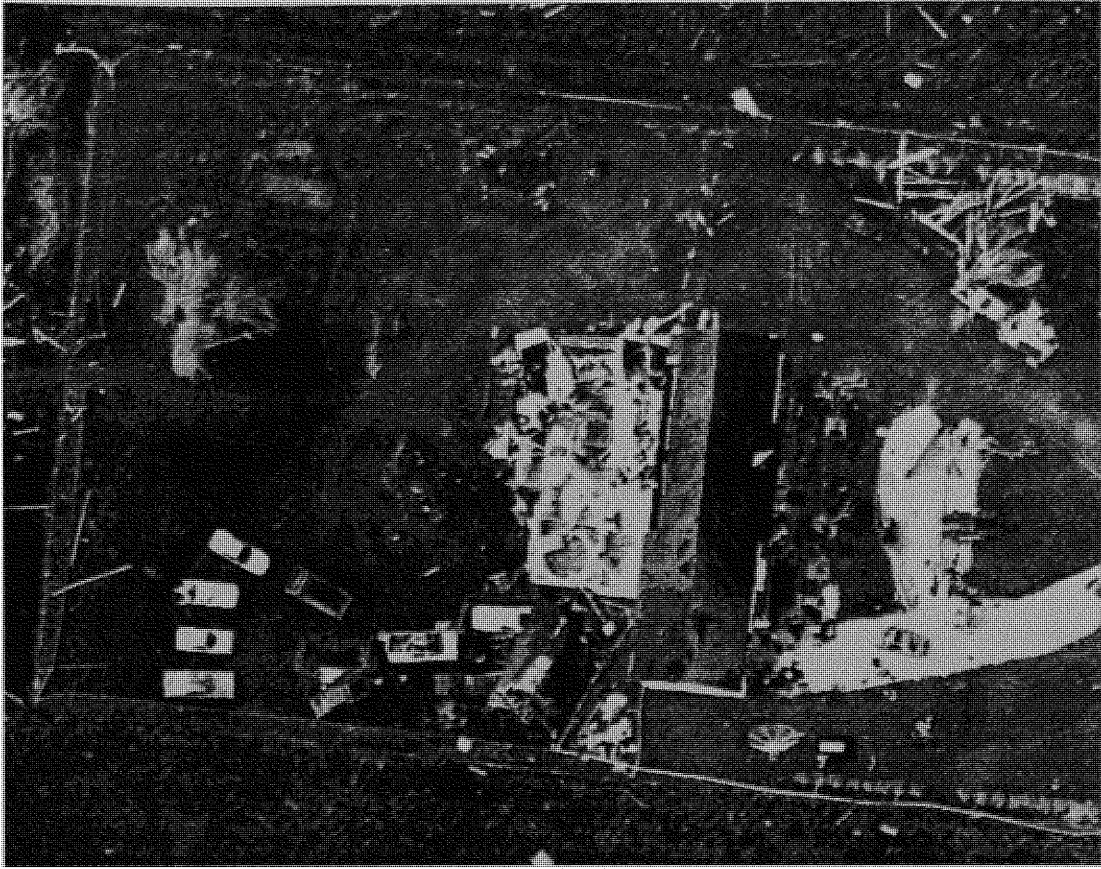
Figure 8.7. Collapsing of main roof structure.
