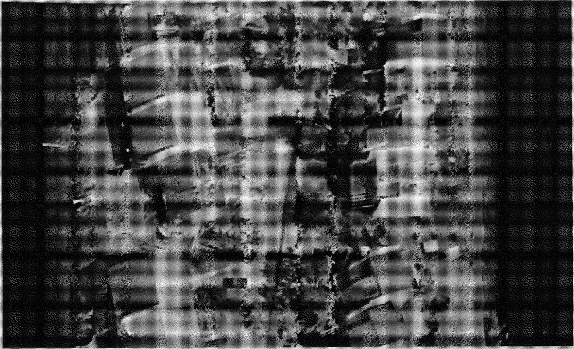
Figure 2.5. Collapsing of roof truss due to saturation load.
