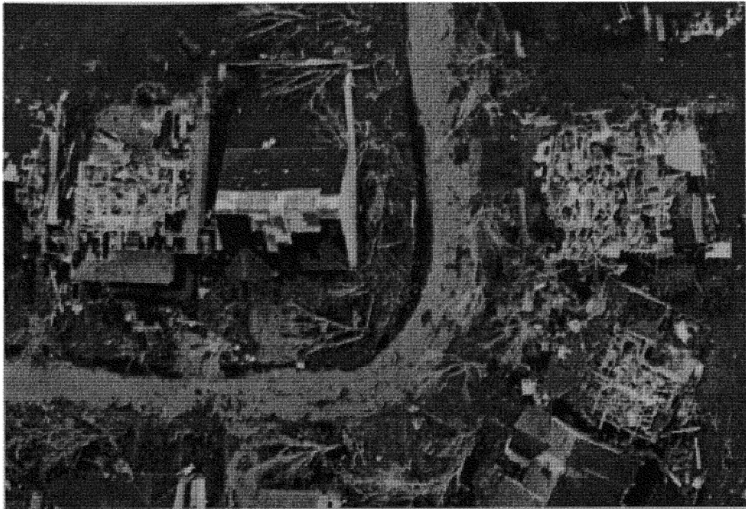
Figure 1.14. Overall damage of 100%.
