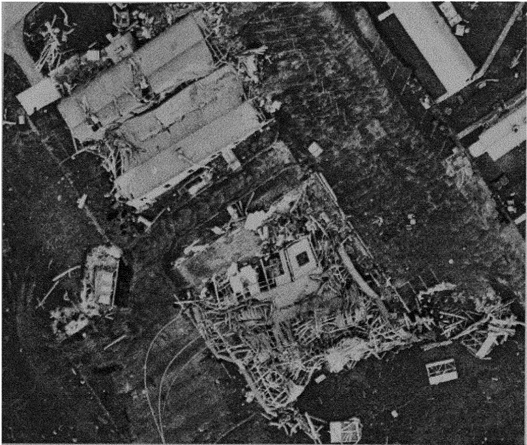
Figure 8.15. Loss of ceiling strength due to water saturation.
