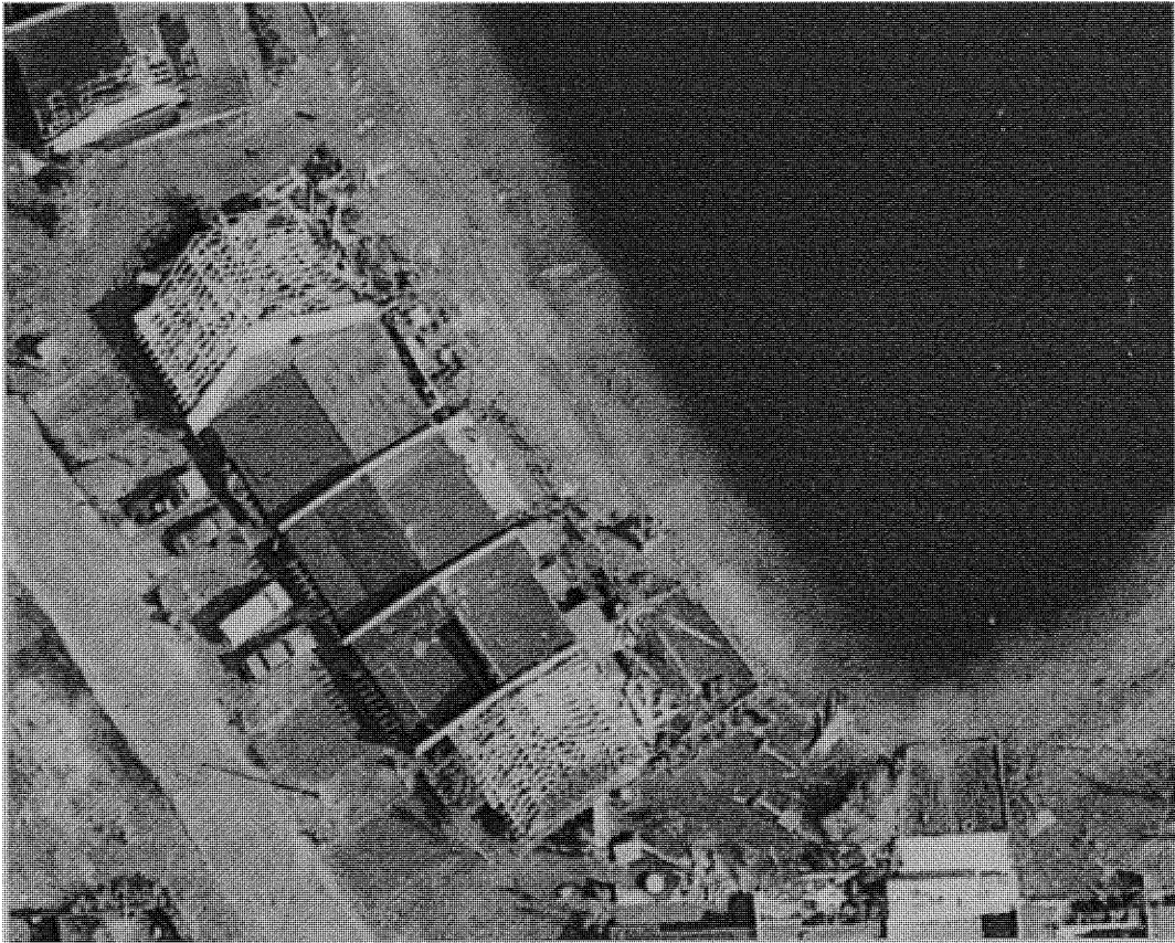
Figure 7.1.5.1. Displacement of trusses.
