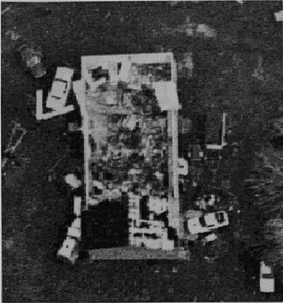
Figure 1.21. Damaged isolated house due to pressurization and depressurization.
