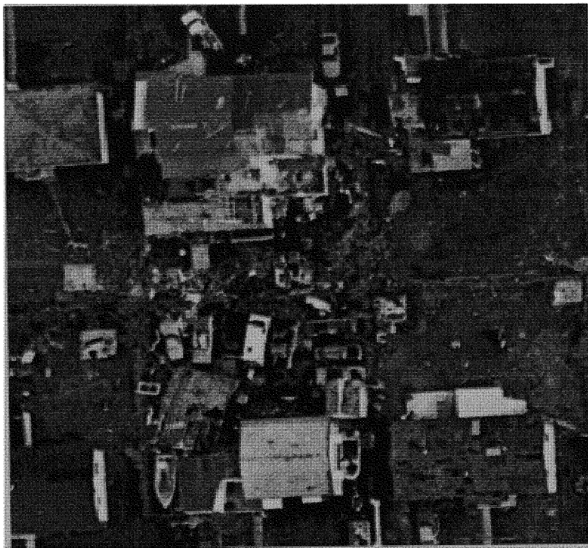
Figure 1.2. Damage due to wind-borne debris.
