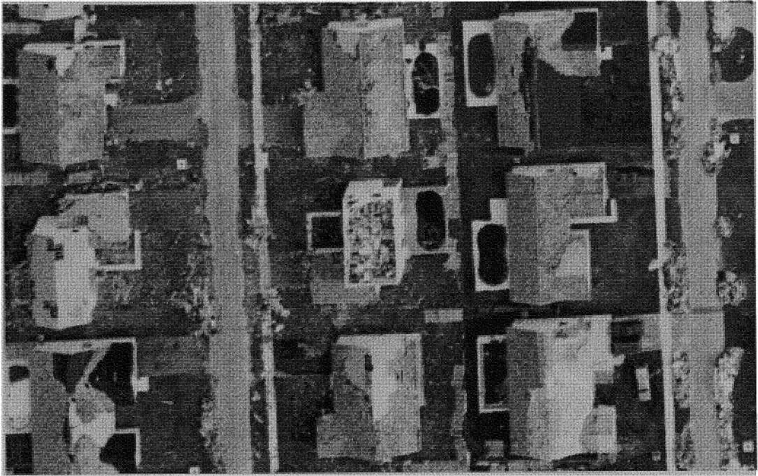
Figure 1.15. Inward collapse of roof trusses.
