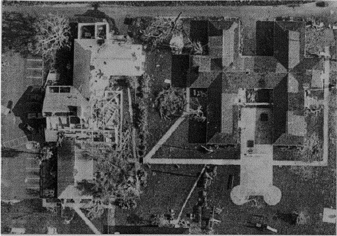
Figure 8.14. Damage to differential roofing system.
