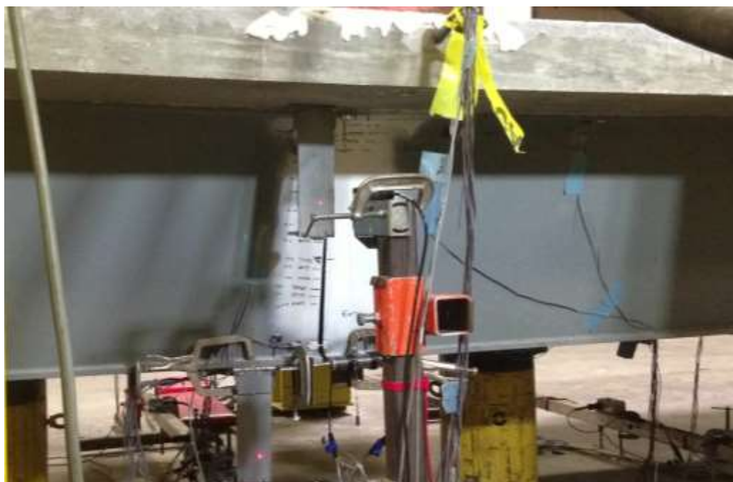
Figure 4-2 East girder with bottom flange and web fractured in one girder.
