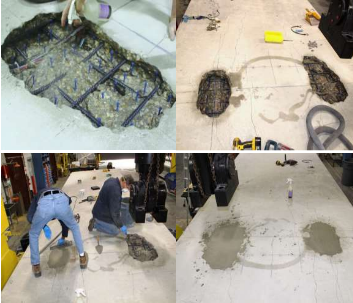
Figure 4-70 Repair of punching shear damage from Tests C and D.
