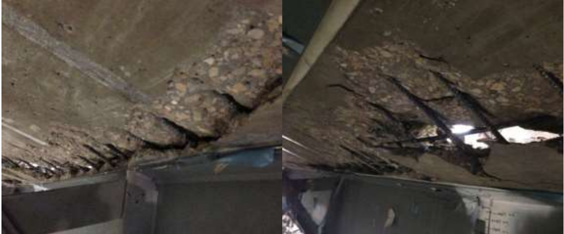
Figure 4-20 Punching in the bottom of the deck.
