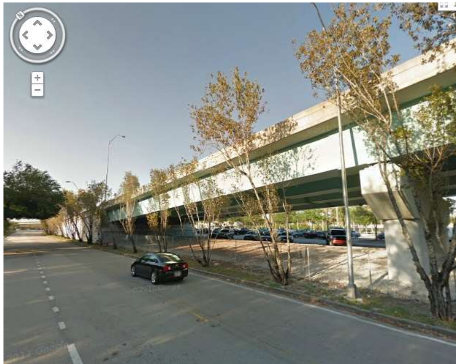
Figure 7-2 First span of the ramp bridge 860600 - elevation view from west.
