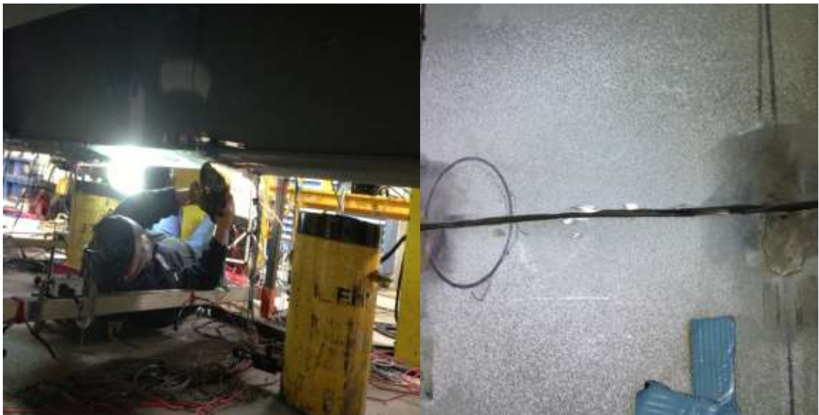
Figure 4-1 Saw cutting of bottom flange in east girder.
