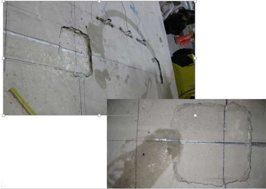
Figure 4-61 Punching damage in Test D.
