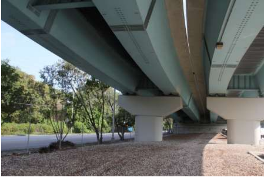
Figure 7-1 First two spans of the ramp bridge - underneath view.
