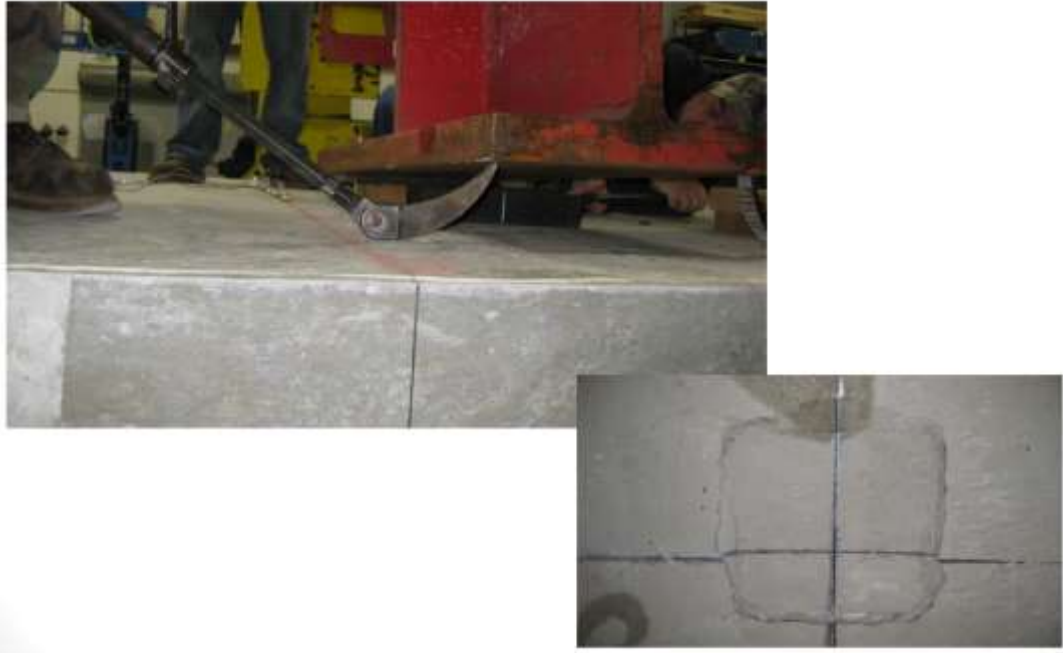
Figure 4-49 Punching damage in test C.
