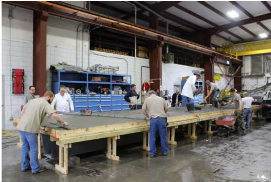
Figure 3-9 Casting the concrete deck.
