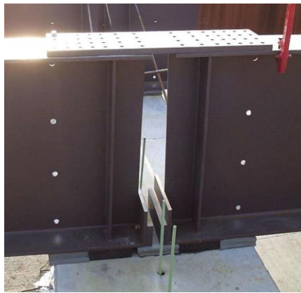
Figure 1-8 Connection detail for Spring Drive bridge.
