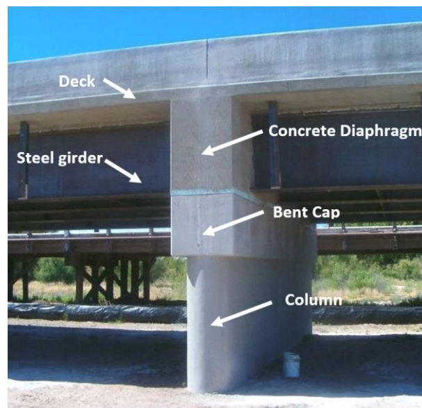
Figure 2-3 Different components of SDCL bridge system.
