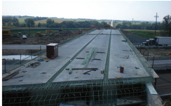
Figure 10-4 Completing the placement of the pre-topped units for the bridge over I-80 at 262nd Street in Nebraska (AZIZINAMINI, 2014).
