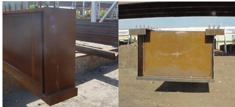
Figure 1-6 Recommended detail for an I girder (left) and a box girder (right).
