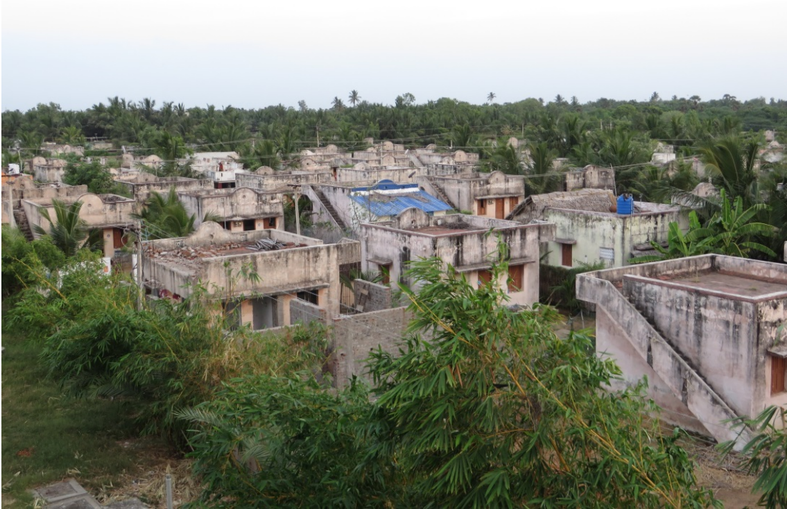
Figure 2. Homes Built After the Tsunami
