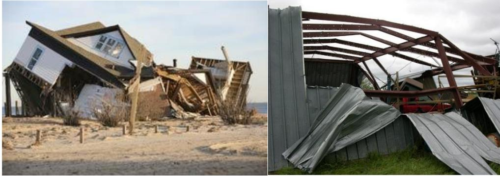
Figure 1.1 Low-rise Industrial Buildings Damaged by High-Wind Events
