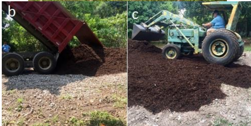
Figure 3: (a) Rototilling grass and surface soil (b) soil delivery (c) leveling out of soil
