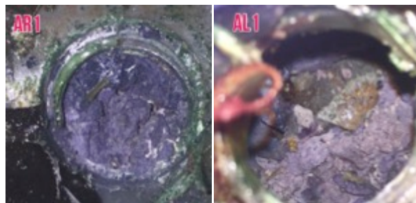
Figure 4.20: Photos of pH Results for the First Corrosion Probe Located at 0.5 ft. from the Top of MIT Test Samples with Zero Additives (A)
