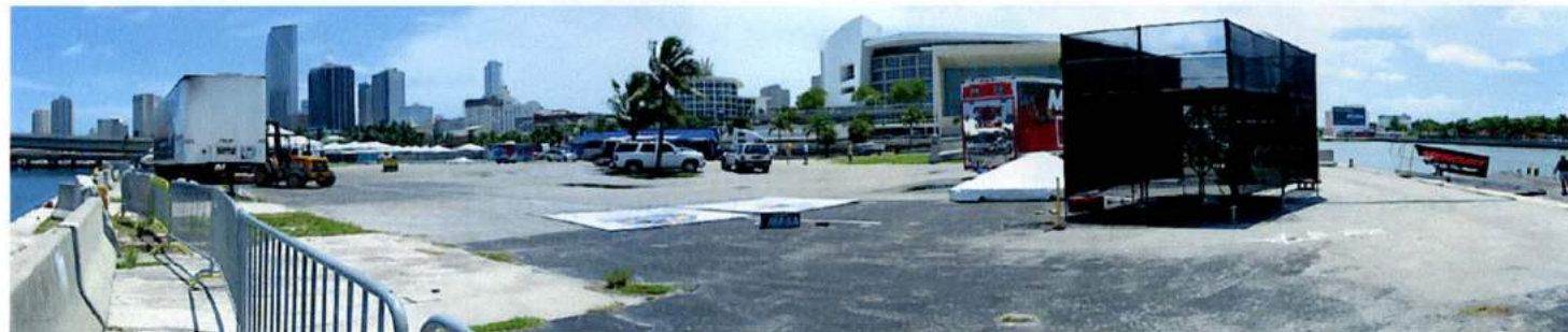
Figure 34. Existing conditions, Parcel B.
