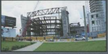
Performing Arts Center (under construction).
