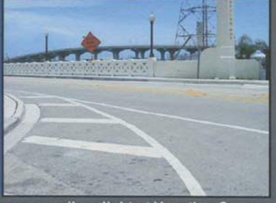
No crosswalk or light at Venetian Causeway.
