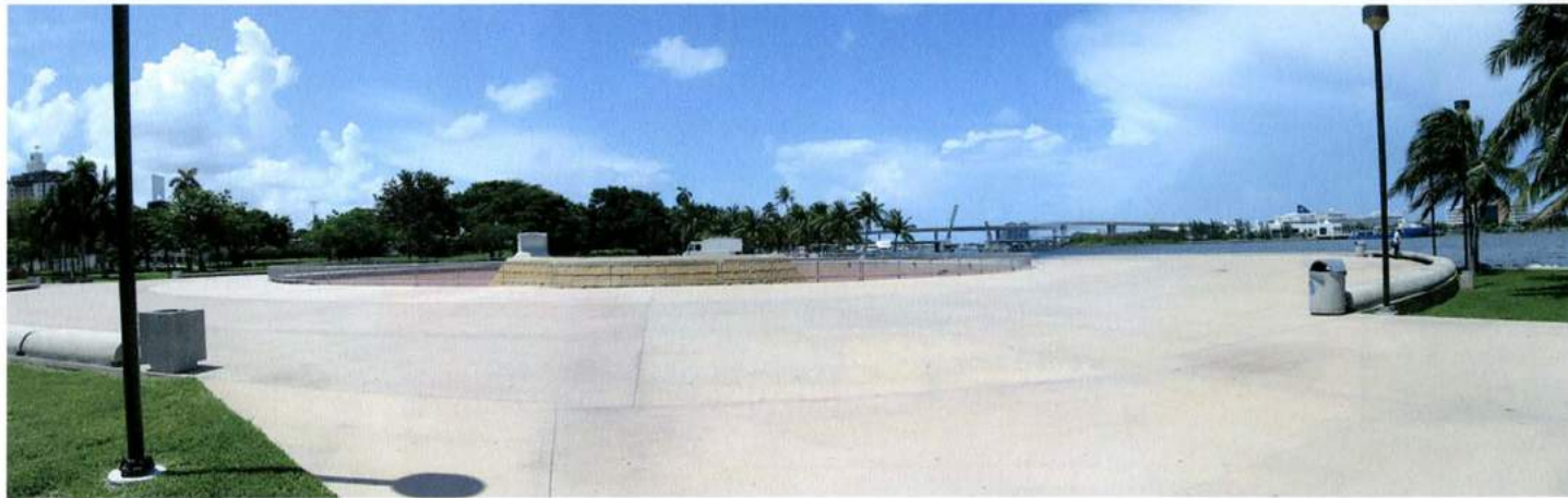
Figure 31. Existing condition of fountain designed by Isamu Noguchi in Bayfront Park.
