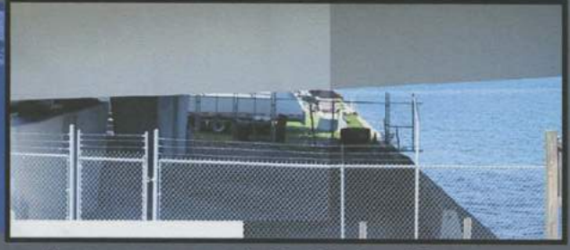
No access over or under Port Boulevard Causeway.
