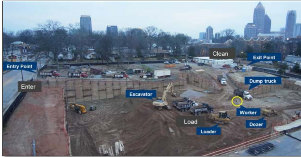
Figure 10: Site Overview (Pradhananga, 2014)
