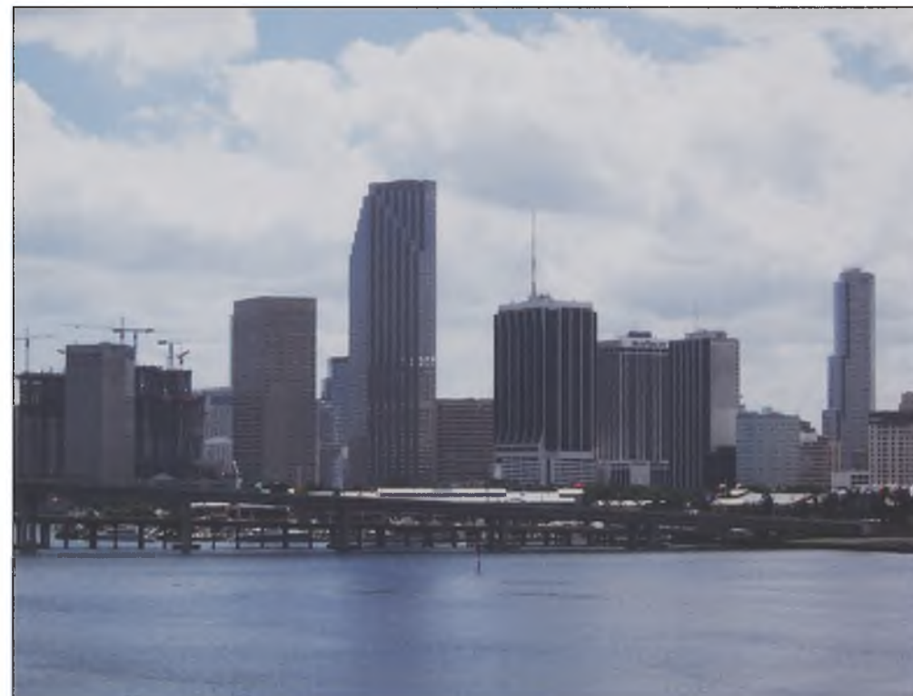
Illustration #30. Site context viewed from the bay
