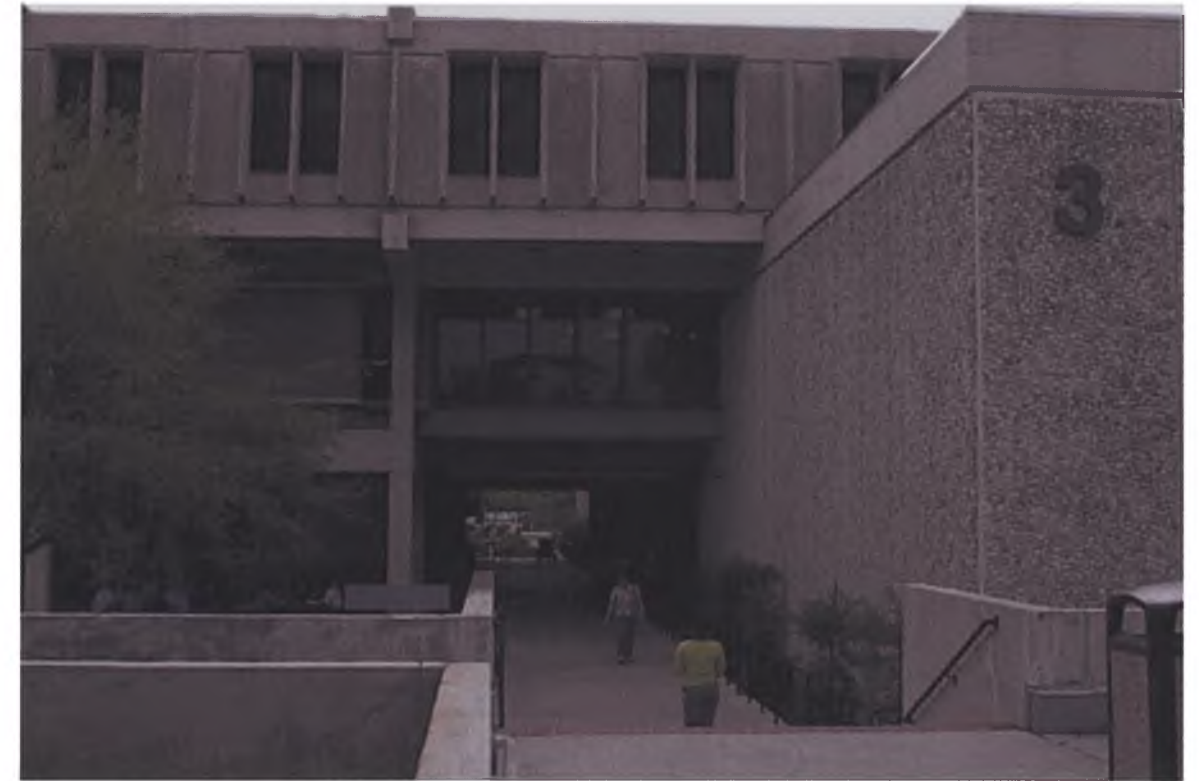
Figure 7 Intersection – MDC. Pedestrian corridors that run through the campus intersect important buildings. Public and private spaces become indistinguishable in the process.
