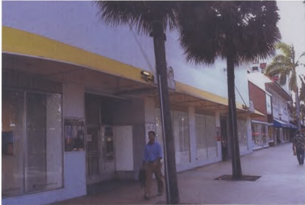
Figure 11 Glass Storefronts – Lincoln Road (AC/SF 810). The typical glass pane openings found on retail storefronts.
