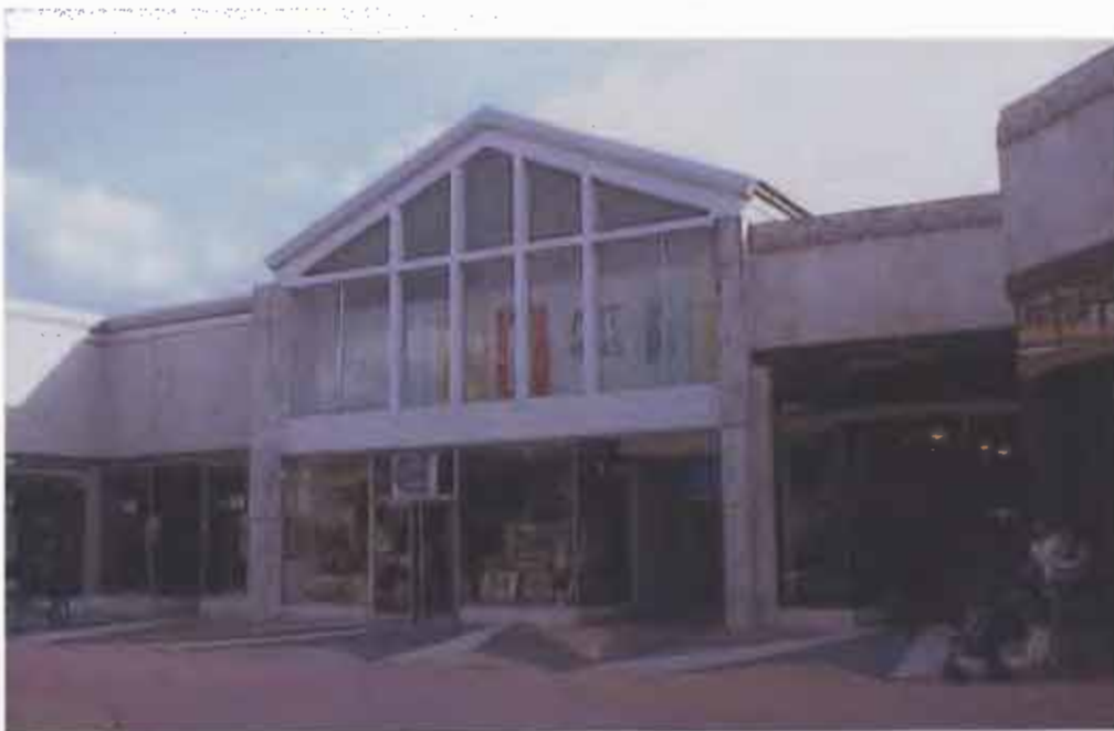
Figure 12 Recessed Entry – Lincoln Road (AC/ SF 924). The facade of the Art Center benefits from an additional recessed gathering area.
