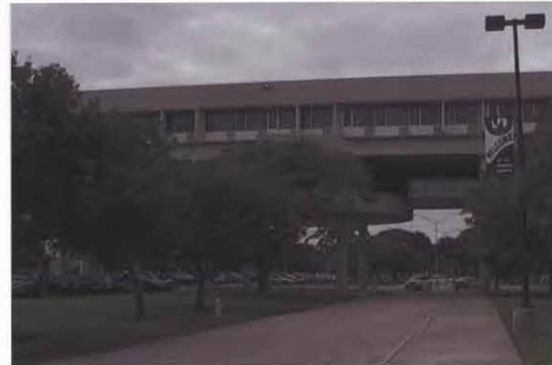
Figure 4 Visual Permeability – MDC (Large Openings). The large opening acts as a gate which visually promotes pedestrian and vehicular traffic access.
