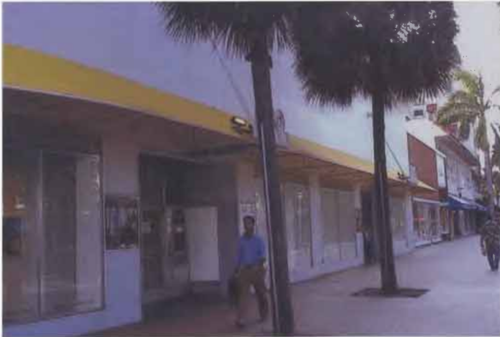
Figure 11 Glass Storefronts – Lincoln Road (AC/SF 810). The typical glass pane openings found on retail storefronts.
