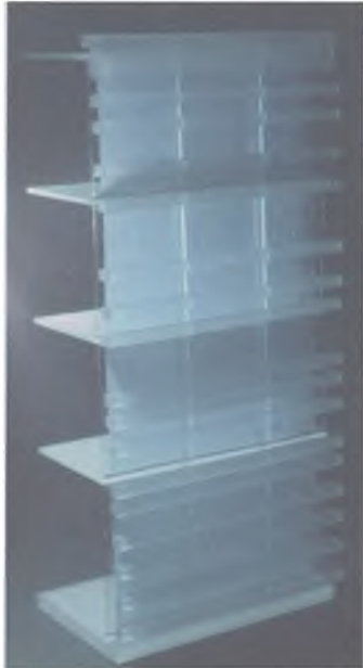
FIGURE 6 6 SECTIONAL MODEL OF EAST CLADDING SYSTEM
