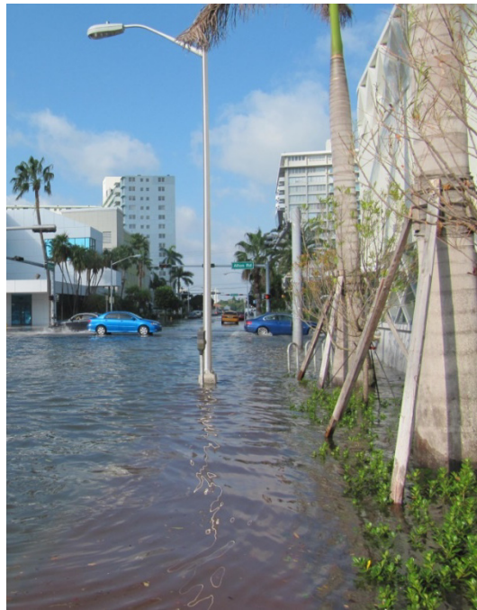
Figure 14: Flooded landscaping, October 28, 2012. Photo by author.
