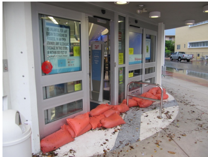
Figure 18: Sandbags Piled in Front of Store, June 8, 2012. Photo by author.
