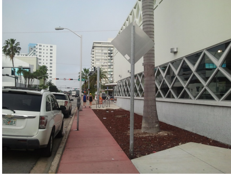
Figure 15: Flood-proofed Landscaping, February 9, 2014. Photo by author.
