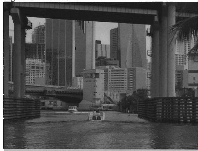
Figure 8 – Site Photo – Miami River
