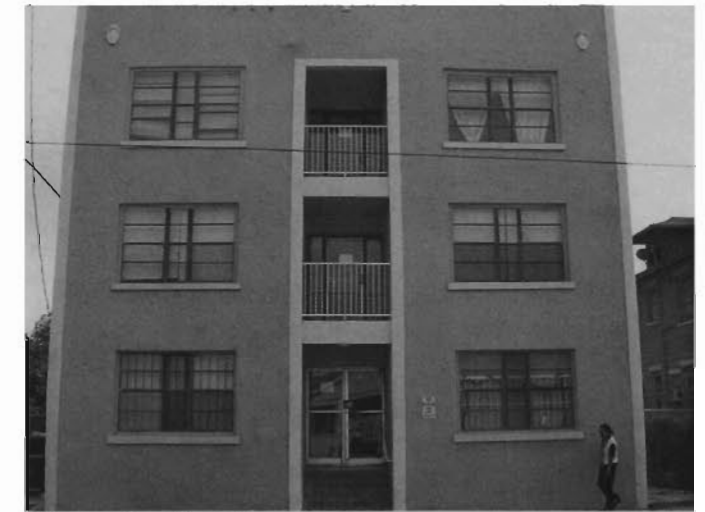
Figure 7 – Site Photo – Medium Density Example
