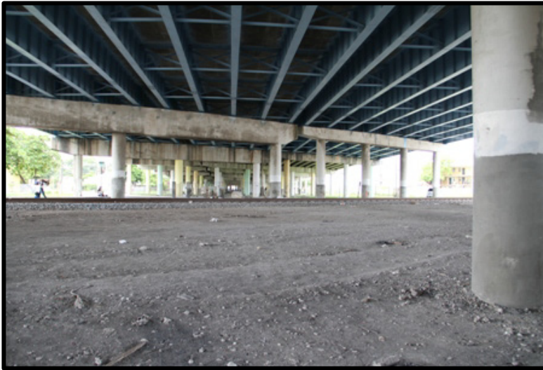
Figure 2: (photo) Under the 395 overpass, downtown Miami
