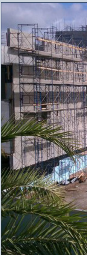
Construction continues at Disney.
