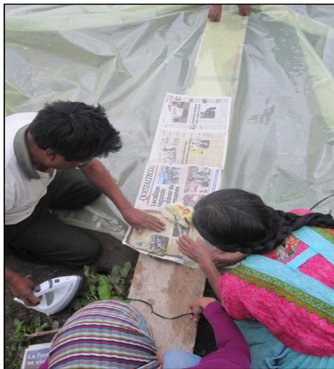
FIGURE 4.2: A POSC PROMOTER (LEFT) ASSISTING MEMBER FARMERS CONSTRUCTING A GREENHOUSE
