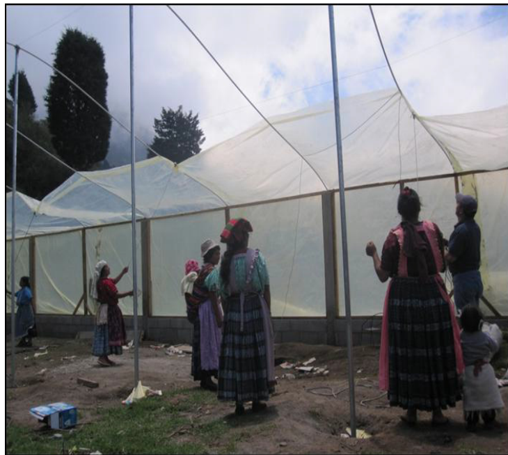
FIGURE 6.4: POSC MEMBERS CONSTRUCTING A GREENHOUSE
