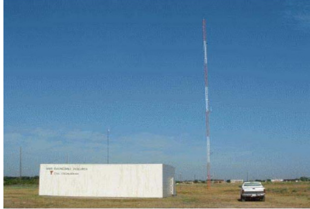
Figure 2.4: TTU Wind Engineering Research Field Laboratory Building
