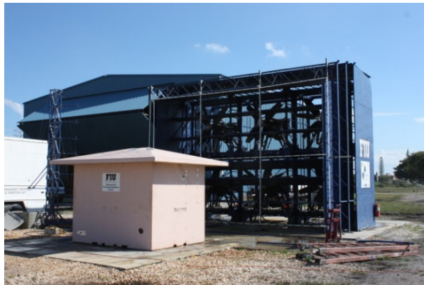
Figure 3.11: Bare Roof Deck
