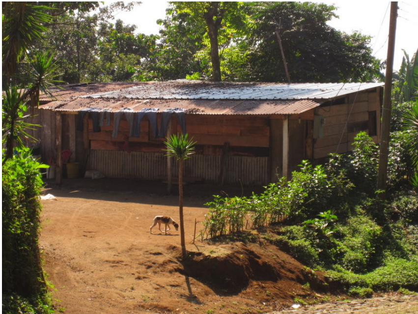
Figure 3.9 La Esperanza: wood plank and corrugated steel type construction is typical of about 25 families in the community
