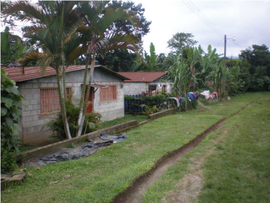
Figure 3.6 Alta Gracia: side-by-side block constructed homes
