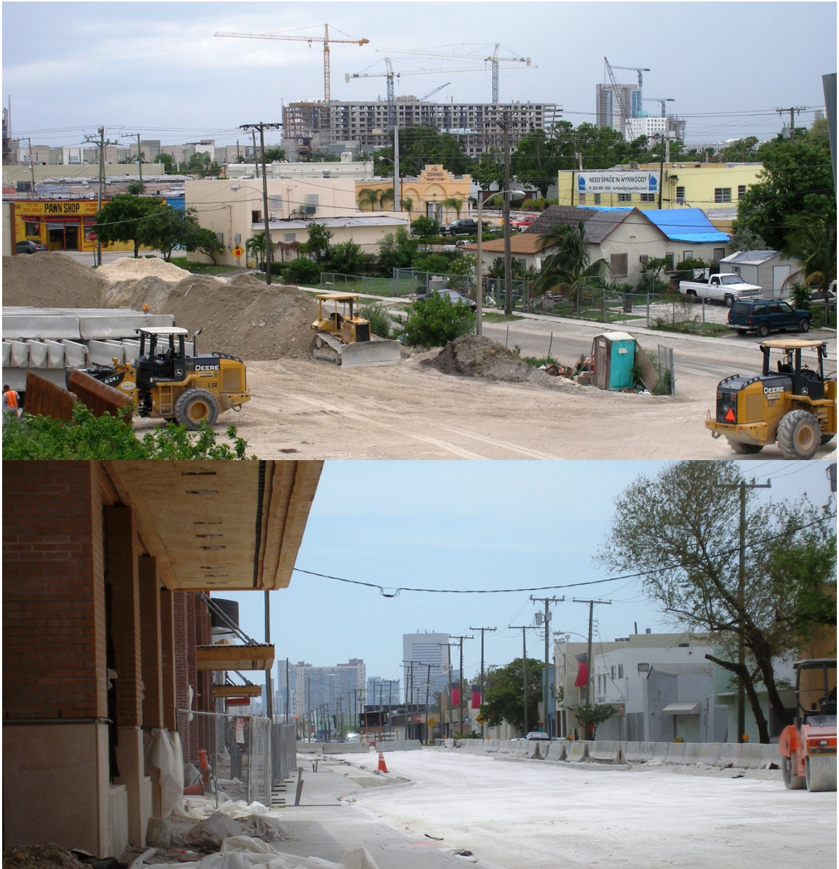
Figure 1.1: Images of Major Construction Transforming Wynwood in 2006
