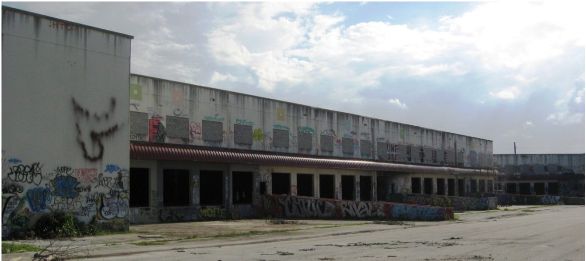
Figure 4.6: Image of the Failed Wynwood Free Trade Zone Site, 2010
