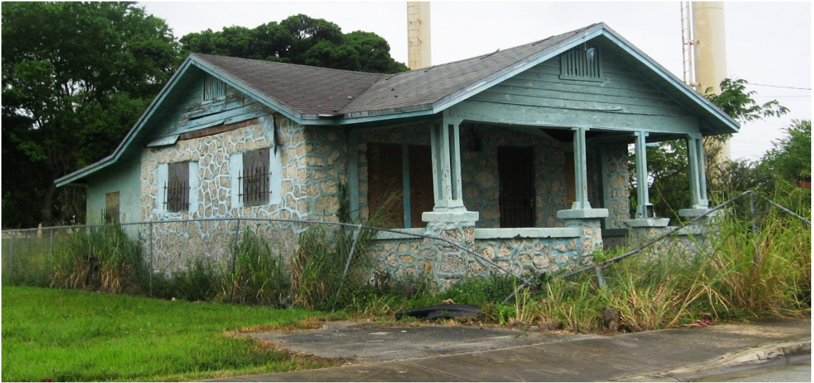
Figure 5.3: Images of Historic Bungalow Homes in Wynwood
