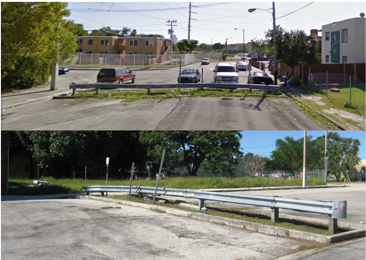
Figure 4.4: Views of Street Closures Along NW 22 Street
