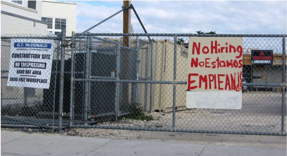
Figure 6:16: Image of a Construction Site with a “No Hiring” Sign in Wynwood
