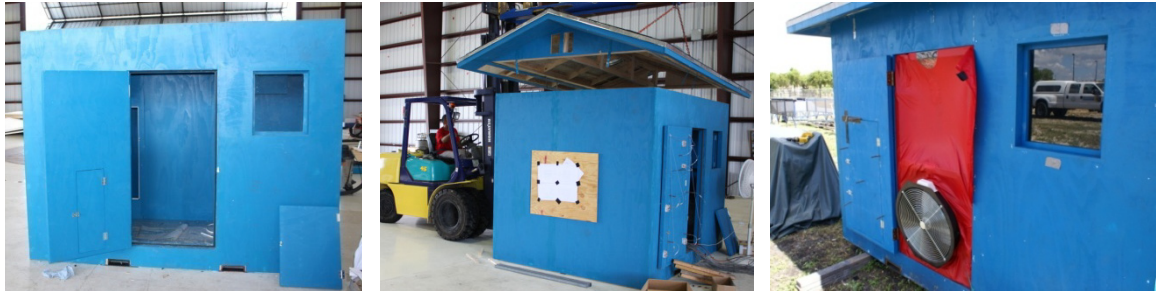
Figure 7.2: Building model from conceptual design to construction, fabrication and door blower test for porosity.
