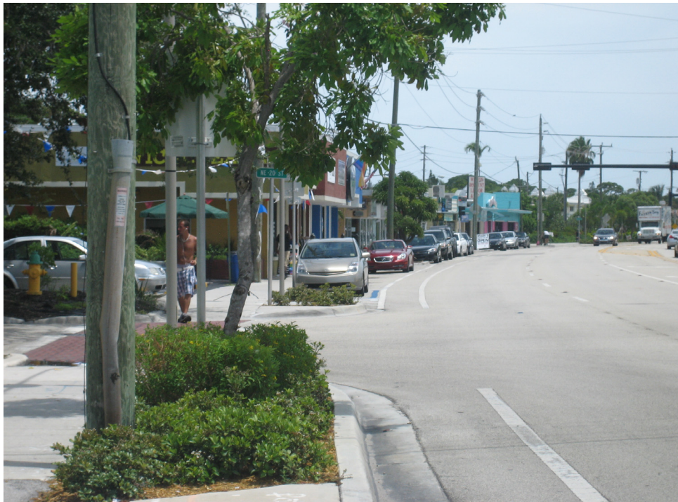
Figure 50. Looking from west to east on Wilton Drive and N.E. 6 th Ave. Photo by Emma Ergon 2011
