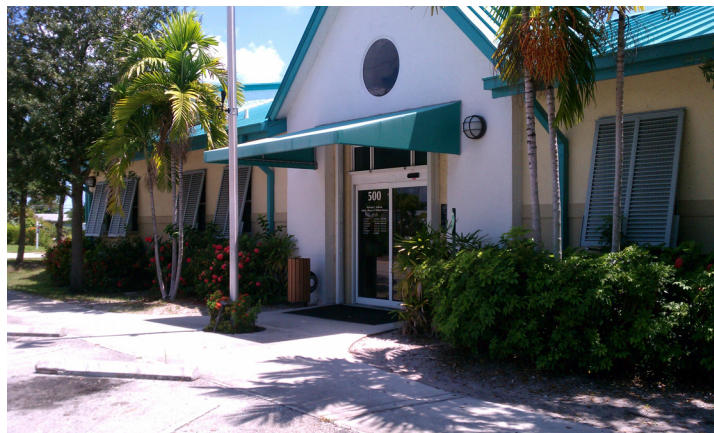
Figure 39. Wilton Manors Library located at northeast 26 th Street. Photo by Emma Ergon 2011
