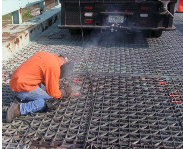
Figure 1.2 Re-Welding of Joints Broken due to Fatigue
