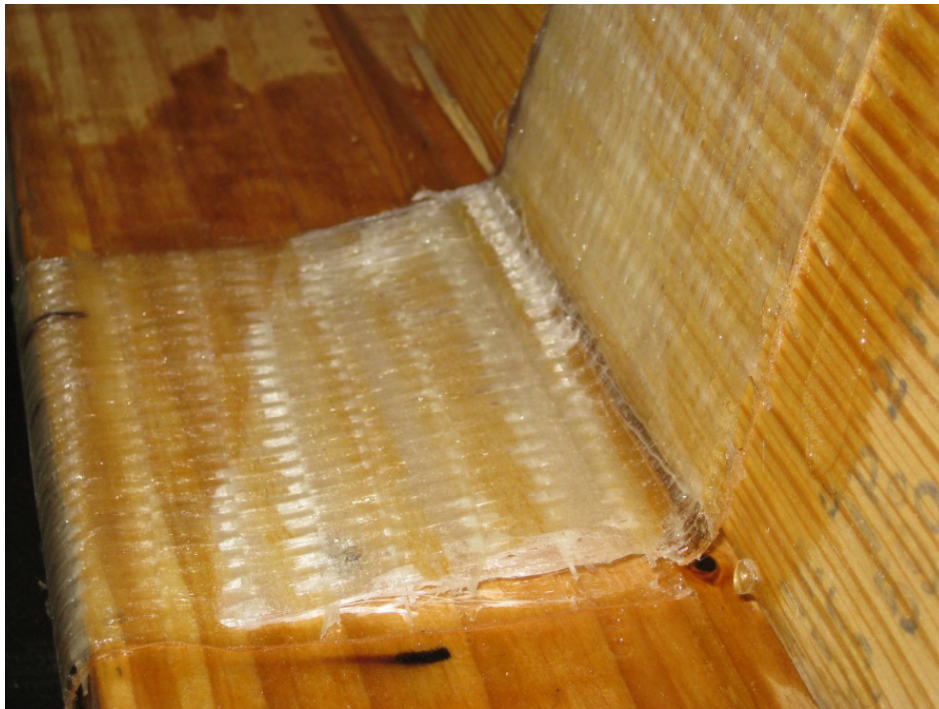
Figure 4-17 Failure mode of configuration-2
