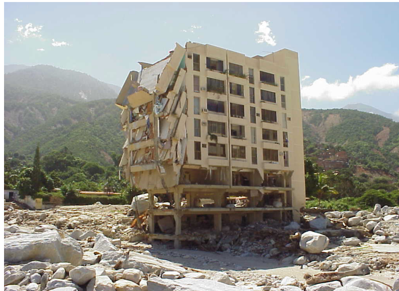
Figure 2. Building destroyed by debris flow; Vargas, Venezuela; December 1999 (Foto R. Garcia, 2000)
