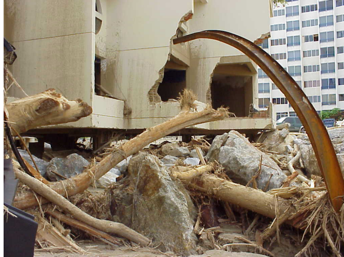
Figure 3. Debris flow deposits around a building, Vargas, Venezuela; December 1999 (Foto R. Garcia, 2000)(Foto R. Garcia, 2000)
