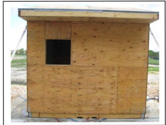
Figure 5.24: Partially Enclosed One Window Removed 90°
