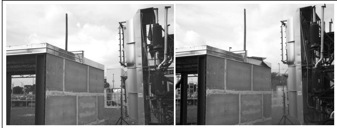
Figure 3.9: Metal Roof Edge Fascia Testing
