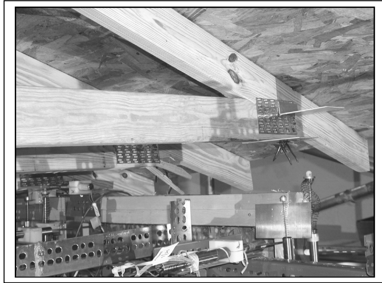
Figure 2.8: Failure of Toe-Nail Connection with a Lateral Load (NIST 2003)
