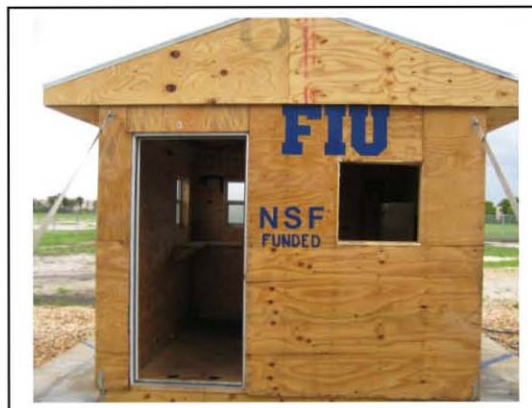
Figure 5.27: Partially Enclosed One Window & Door Removed 0°
