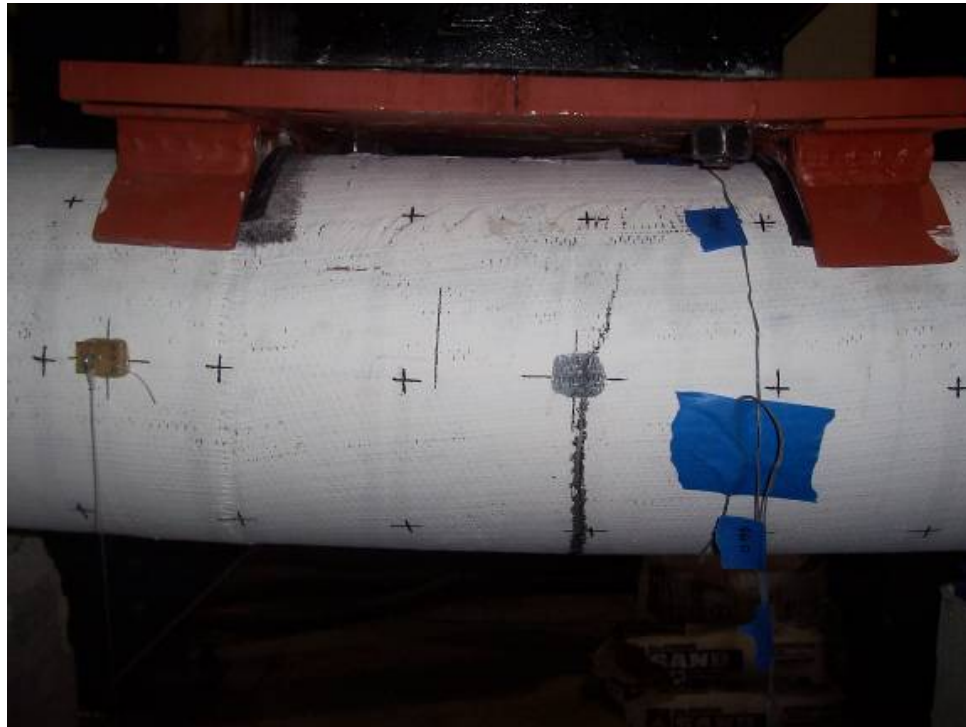
Figure 4.24 Flexural Crack in Specimen SC (West View)
