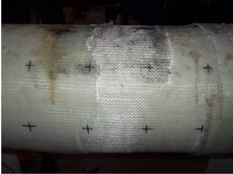
Figure 4.17 Cracking Pattern of Specimen G (West View)
