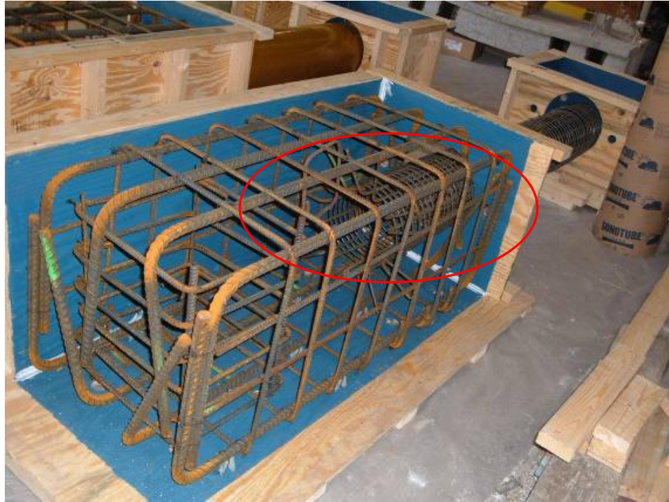
Figure 3.4 Column Reinforcement of Specimen RC Embedded into the Footing
