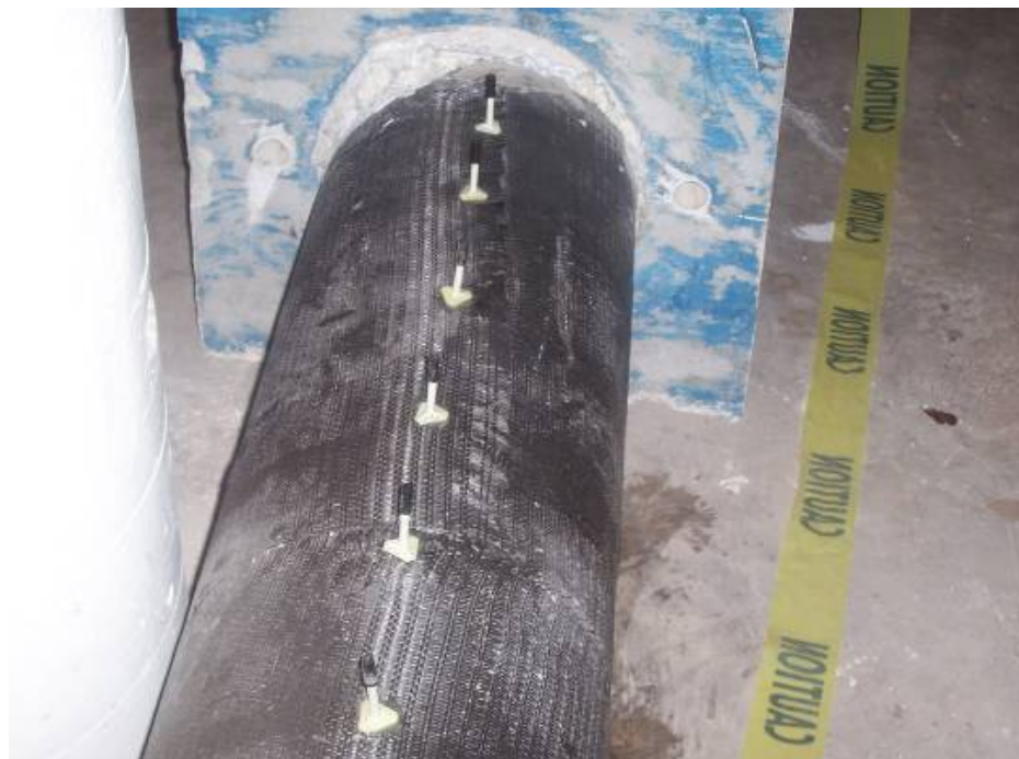
Figure 3.19 Specimen after Epoxy Injection
