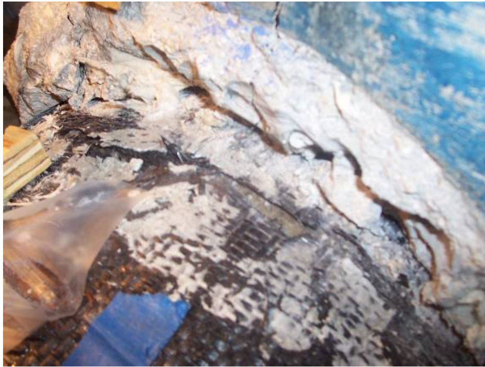
Figure 3.33 Top Fiber Crack in Specimen LC
