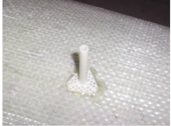
Figure 3.16 Epoxy Injection Port
