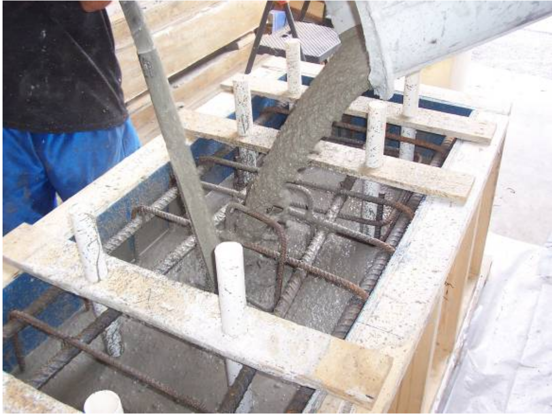
Figure 3.11 Casting of Concrete
