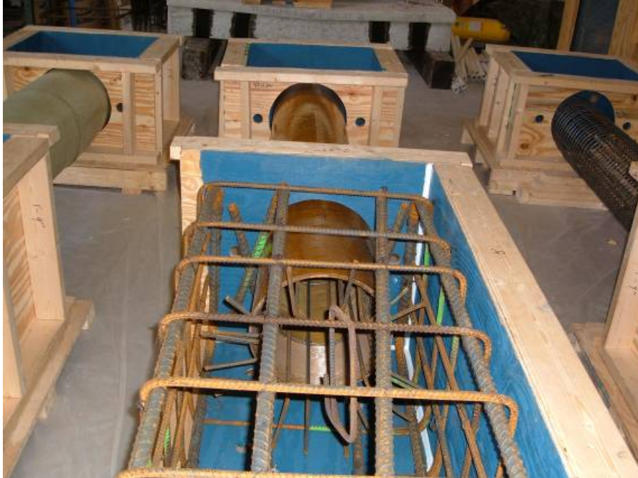
Figure 3.7 Embedment of FRP Tube and Column Reinforcement into the Footing of Specimen Y
