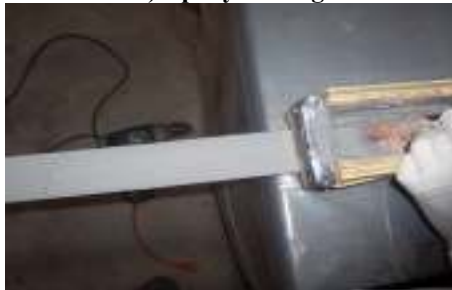
e) Epoxy Applied on the Laminate
