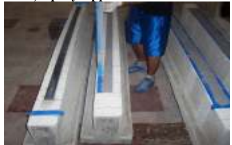
f) Laminate Placed and Tapes Removed
