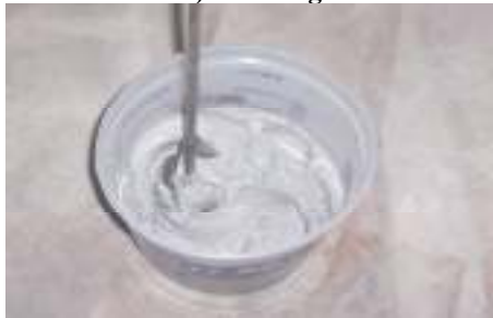
c) Epoxy Mixing
