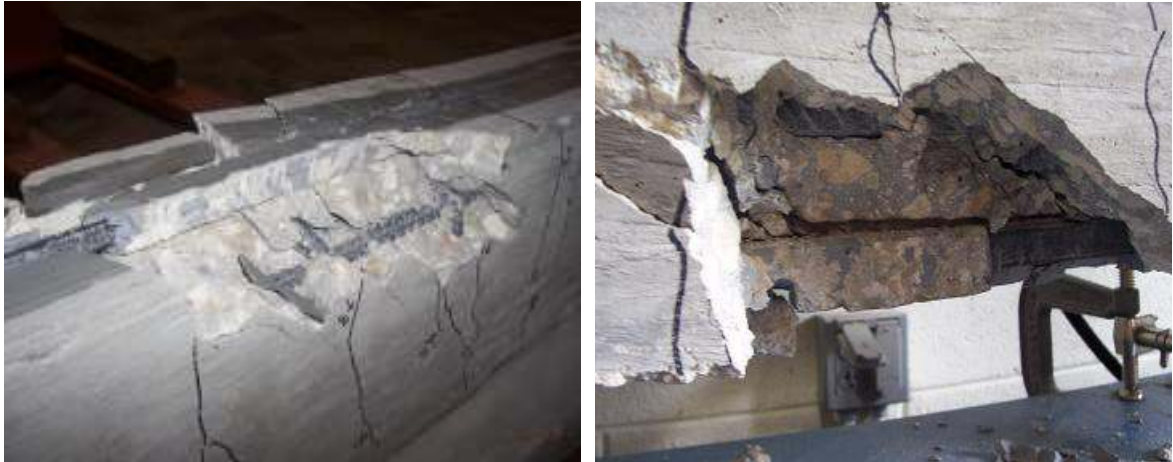
Figure 3.68 Failure Mode of Oversized Specimens (NSM Strip)
