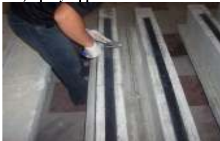
g) Rolling to Ensure No Air Entrapment
