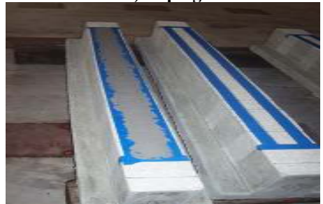
d) Epoxy Applied on the Beams
