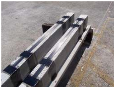
Figure 3.15 Surface Crack Beams Prior to Testing
