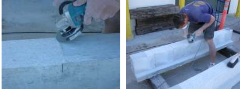
Figure 3.10 Surface Flatness Preparation by Grinding
