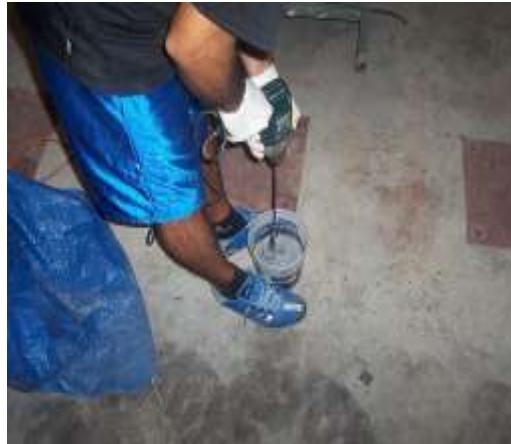
(a) Epoxy Mixing
