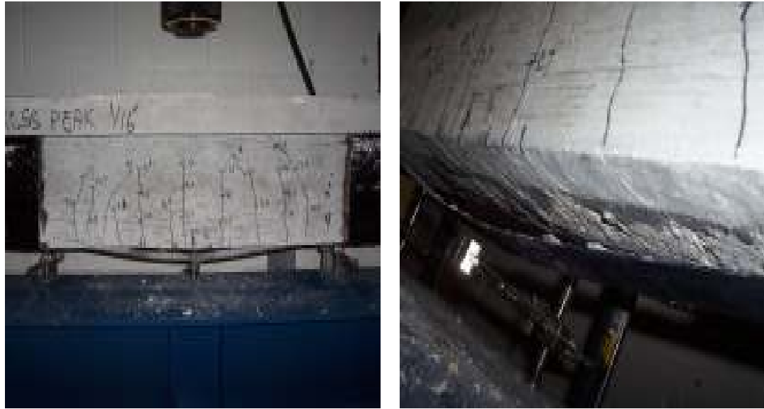
(a) General View (b) Debonded Laminate and Beam Soffit
