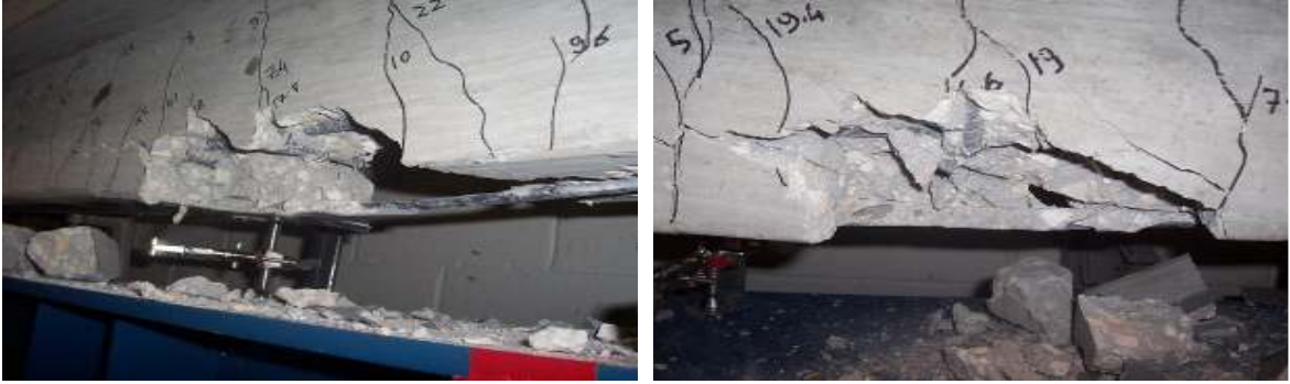
Figure 3.73 Failure Mode of Control Specimens (NSM Bar)
